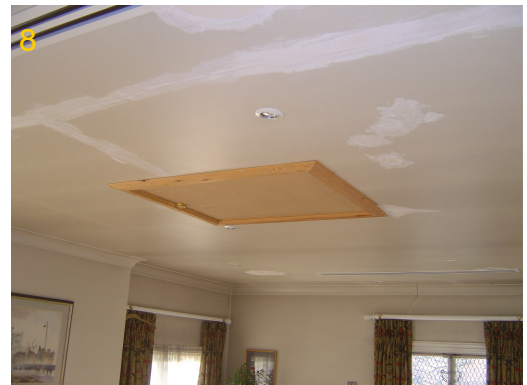
F1.4 LOFT ACCESS TO BE PROVIDED ELSEWHERE AND CEILING RE-INSTATED
