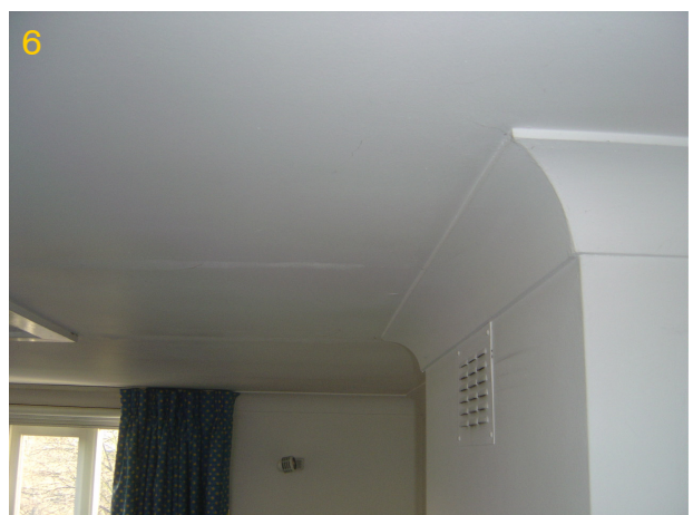
S3 IT IS PROPOSED TO INSTALL BOOKSHELVES EITHER SIDE OF CHIMNEY BREAST AND RE-ALIGN CORNICE TO RUN ALONG TOP OF BOOKSHELVES
