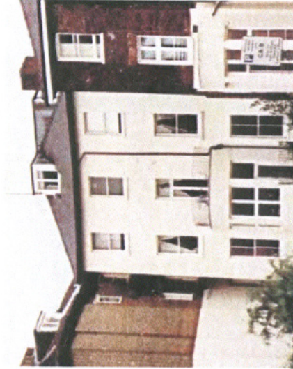
PHOTO 5 Rear facade of 41 Belsize Park as existing. Existing rear dormer is offset in relation to windows below.
