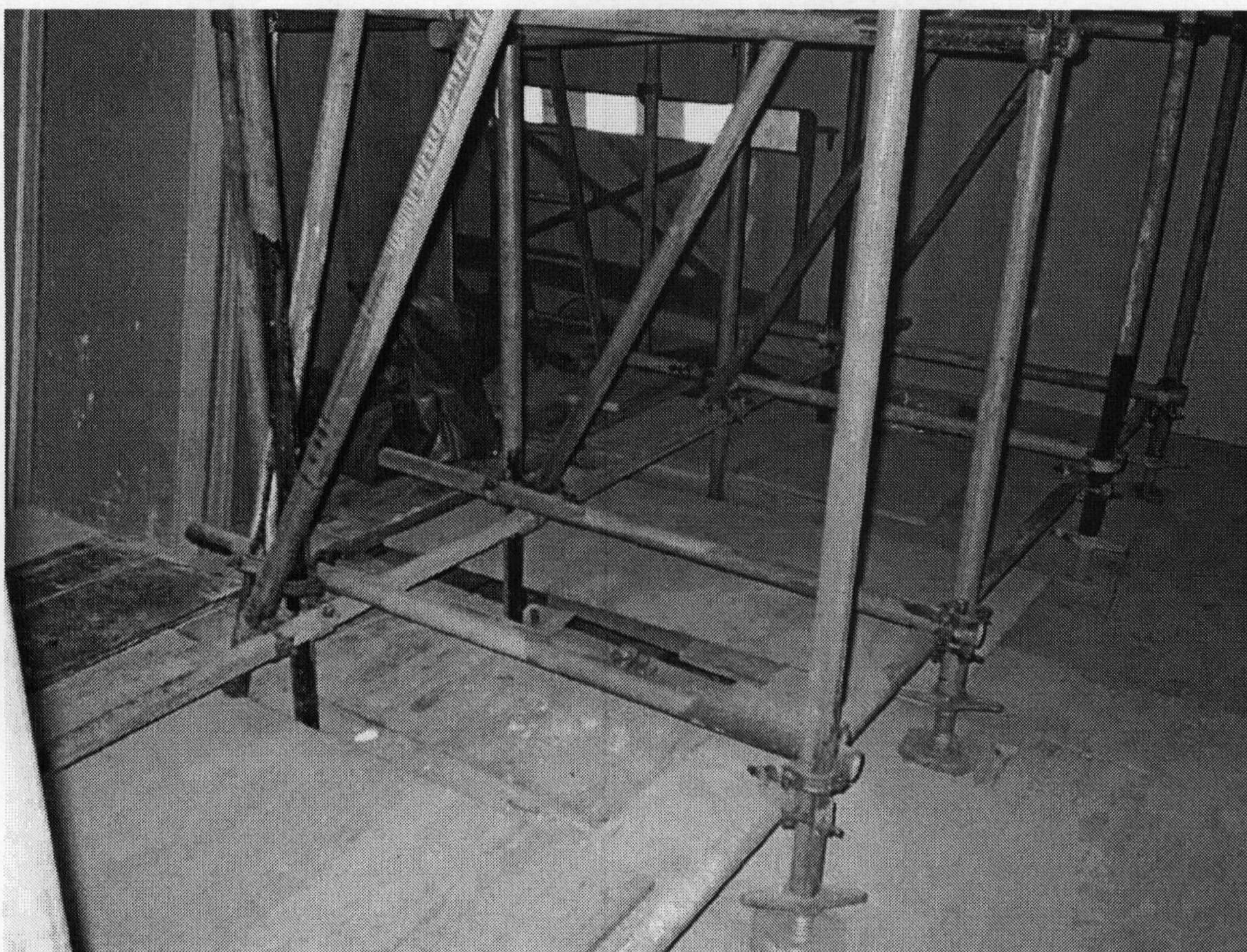
Photograph 8 Gallery 36 Crash deck supported off modern steel beams in floor
