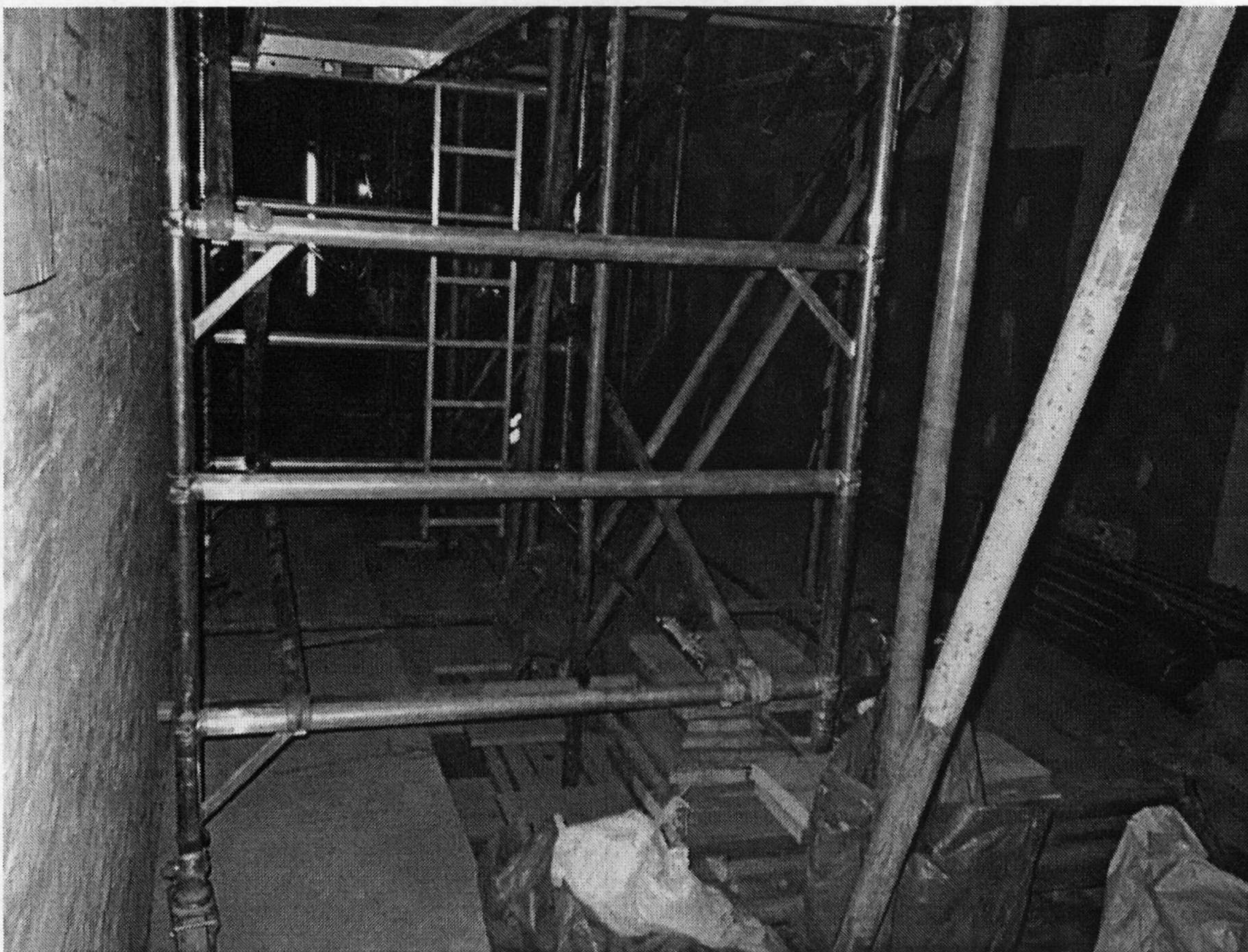
Photograph 3 Gallery 40 South Wall Crash Deck built off modern steel beams spanning across Gallery
