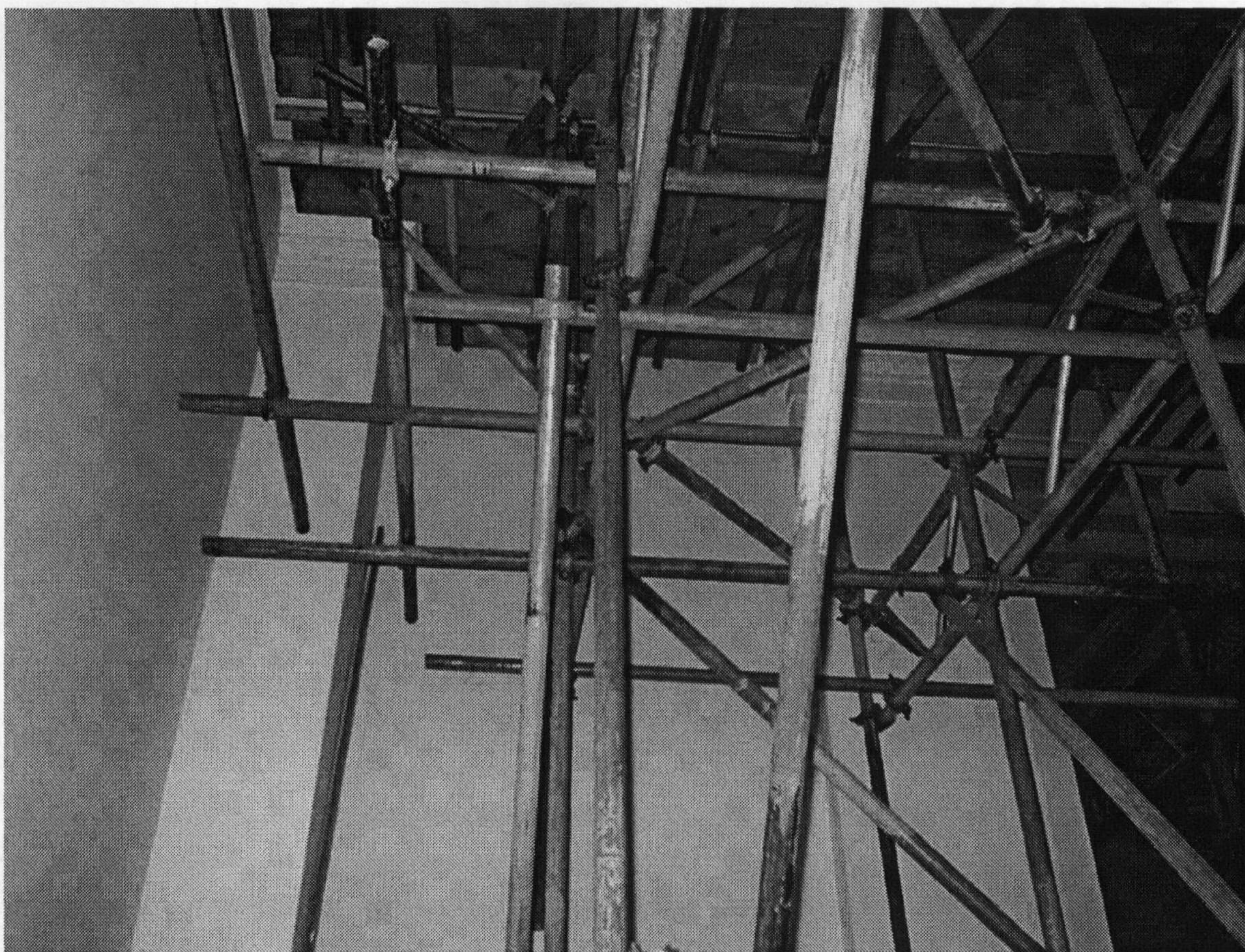
Photograph 7 Gallery 36 South West Corner
