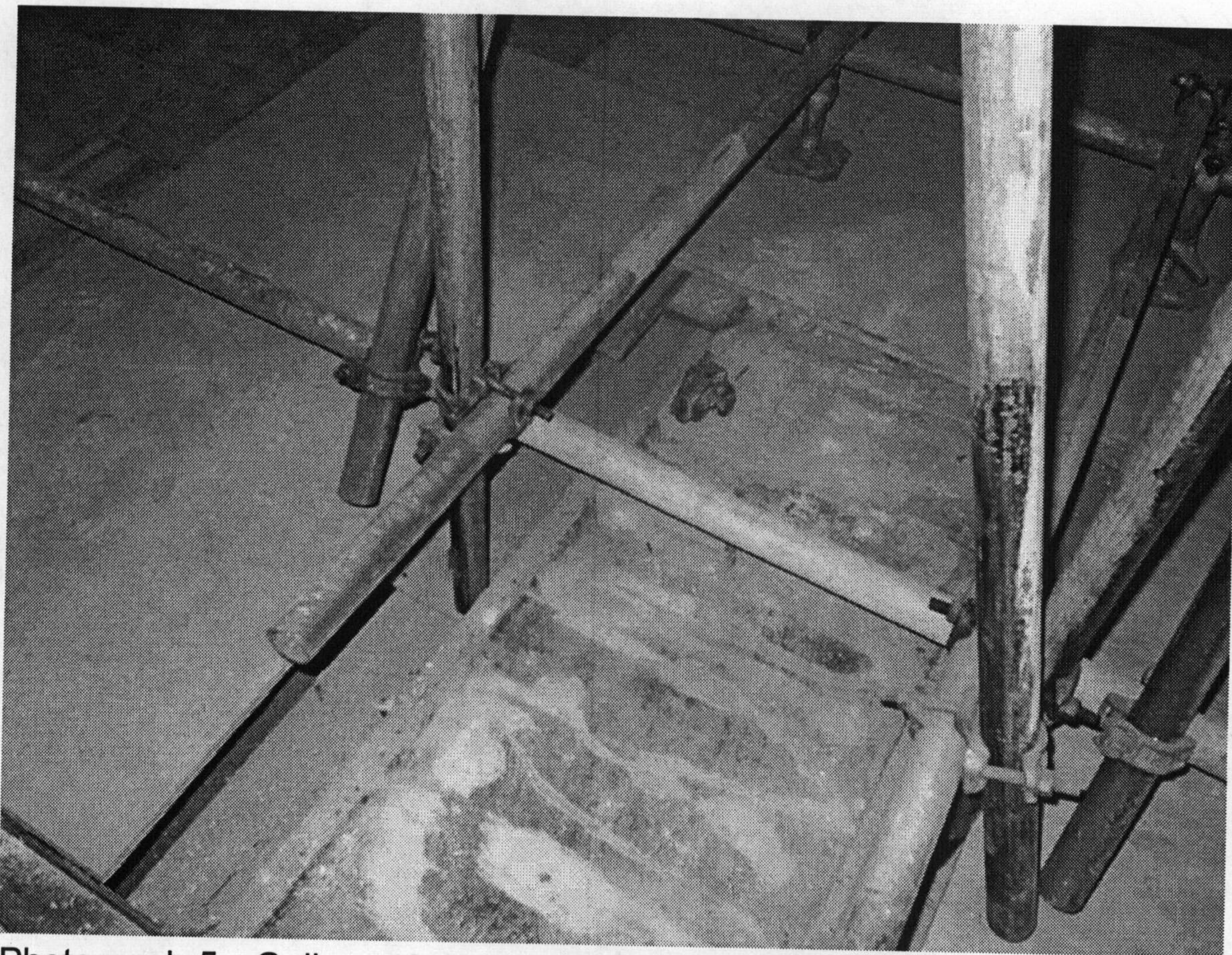
Photograph 5 Gallery 40 Crash deck supported off modern steel beams ( with red paint finish )
