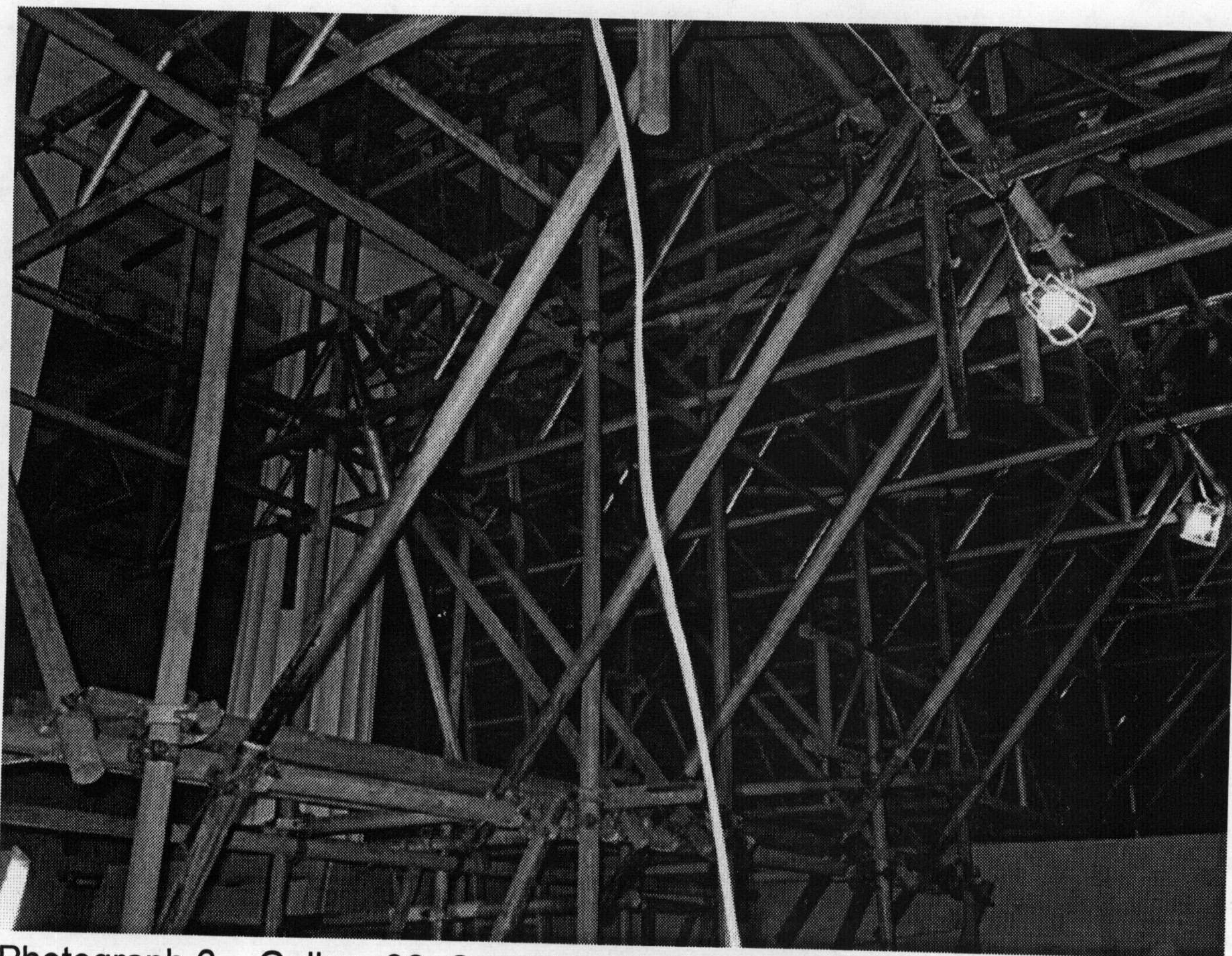
Photograph 5 Gallery 40 Crash deck supported off modern steel beams ( with red paint finish )
