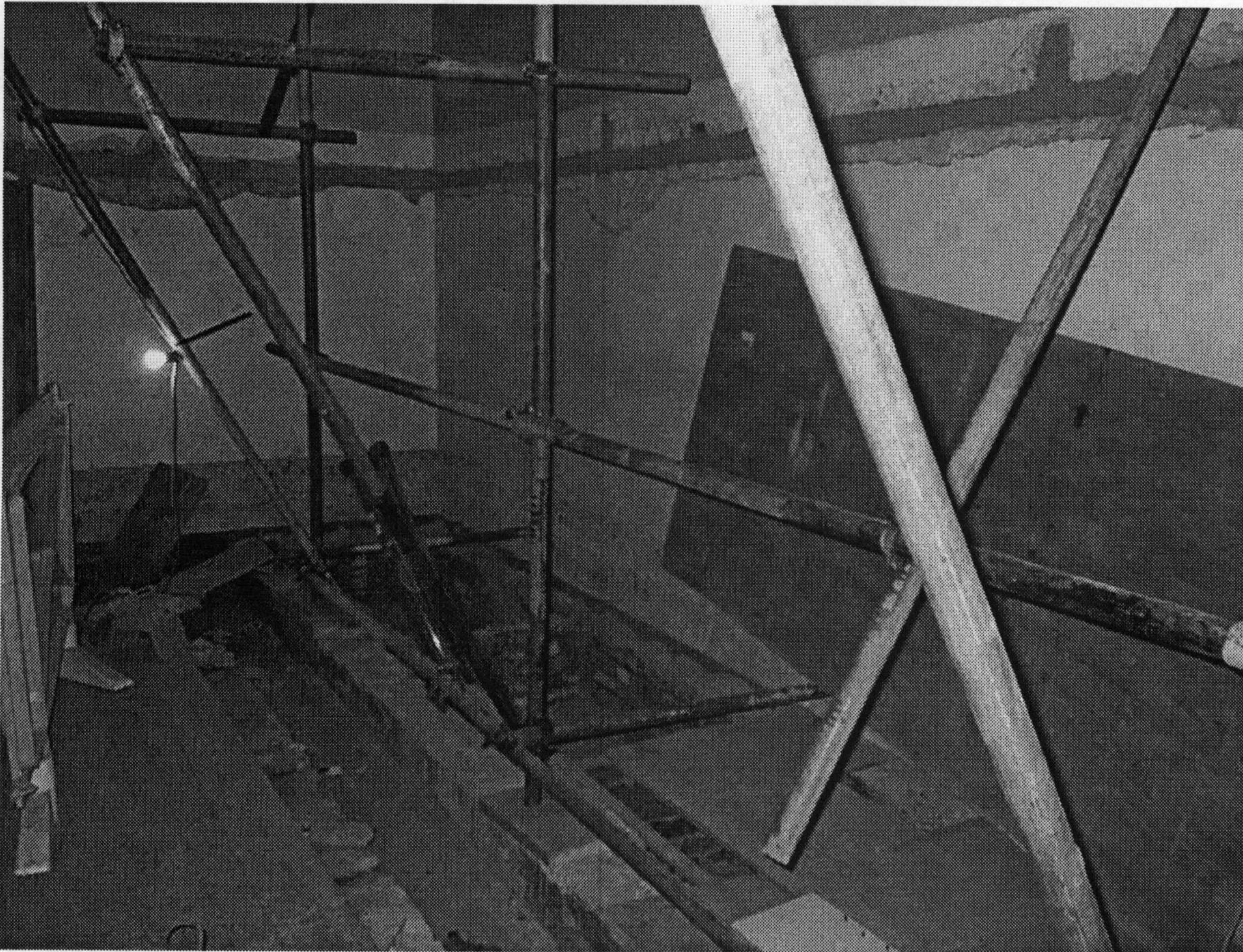
Photograph 1 Gallery 39 Crash deck built off sleeper walls below floor level
