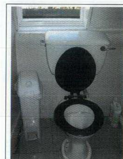
Basement WC 10 Gower Street
