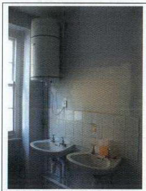
Second Floor WC 12 Gower Street
