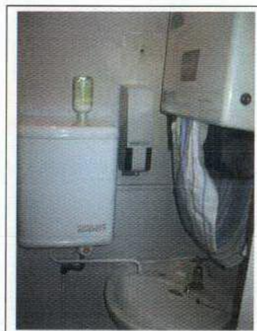
Basement WC 10 Gower Street
