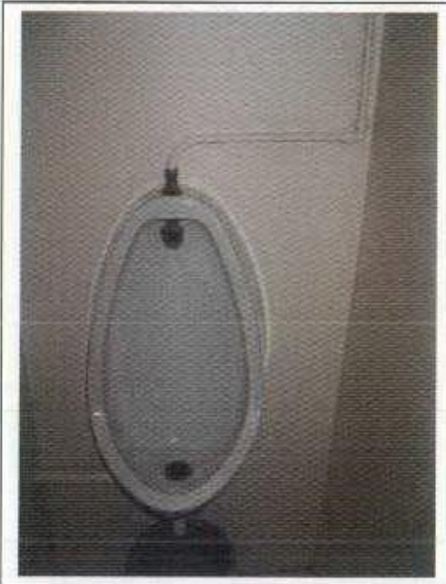
Basement WC 16 Gower Street
