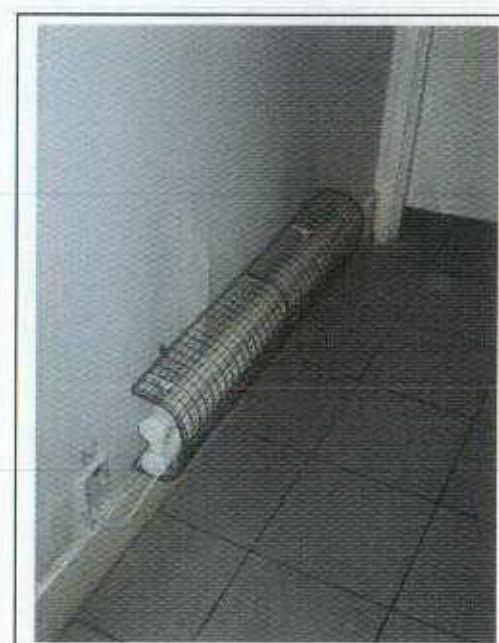
Basement WC 10 Gower Street
