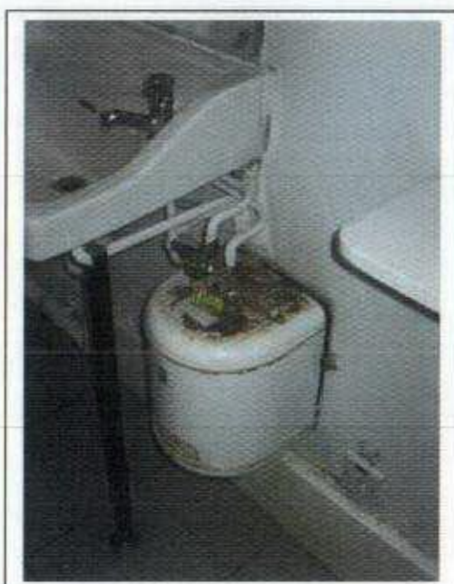
Basement WC 10 Gower Street
