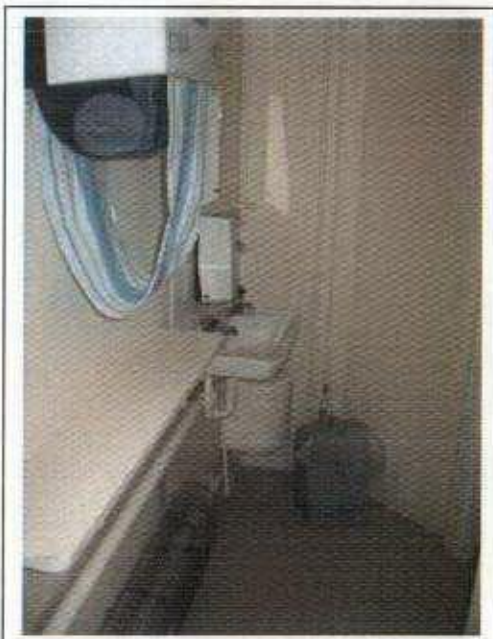
Basement WC 16 Gower Street
