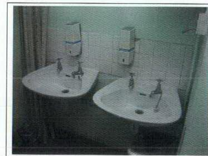
Basement WC 12 Gower Street
