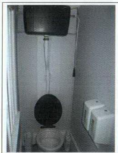
Basement WC 10 Gower Street
