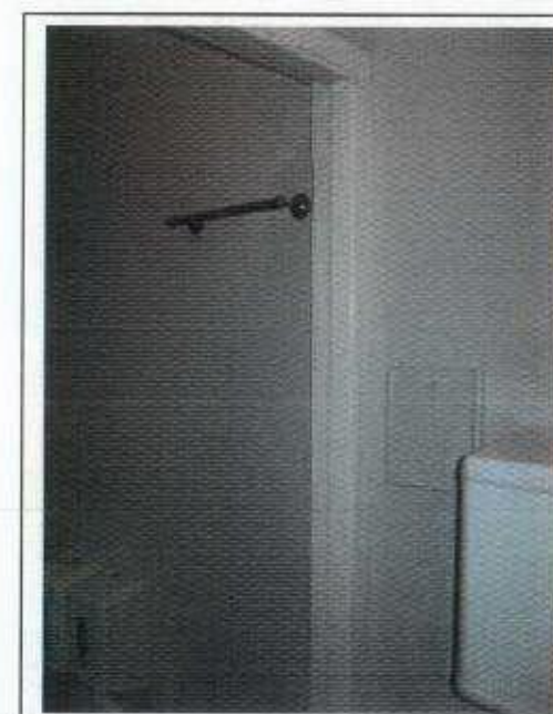
Basement WC 10 Gower Street
