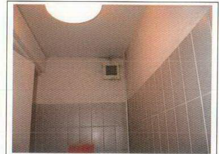
Basement WC's 14 Gower Street
