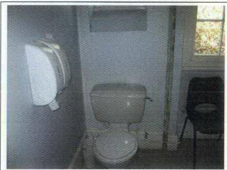
Second Floor WC 12 Gower Street
