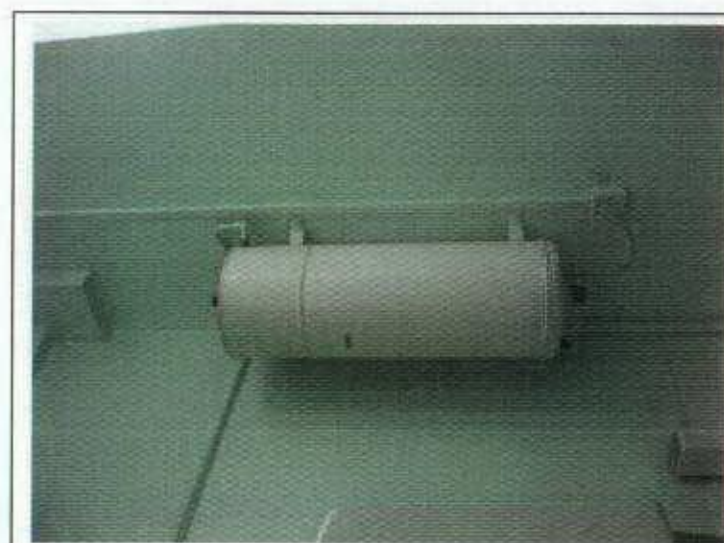
Basement WC 12 Gower Street
