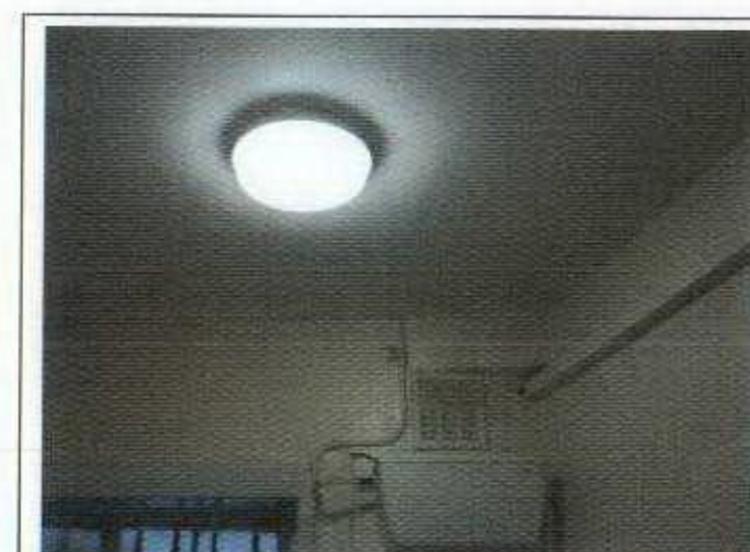
Basement WC 4 Gower Street
