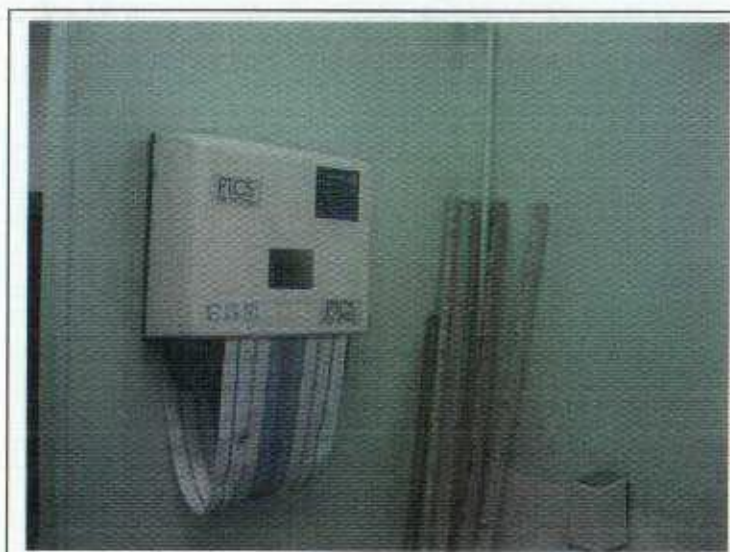
Basement WC 12 Gower Street
