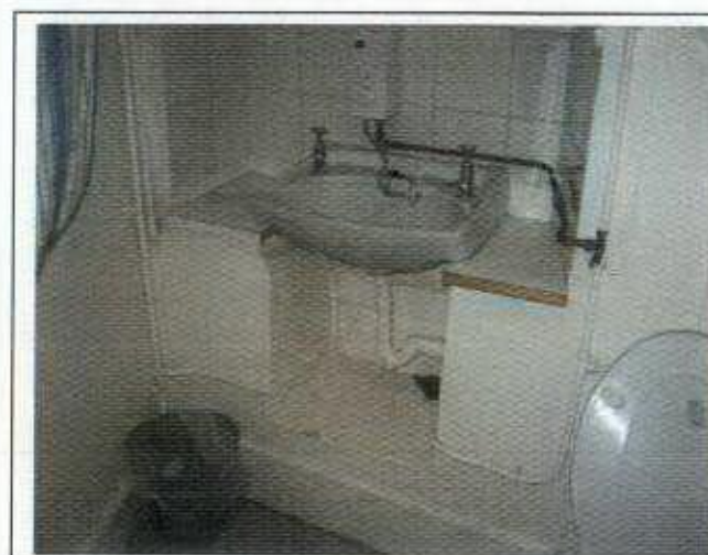
Basement WC 4 Gower Street
