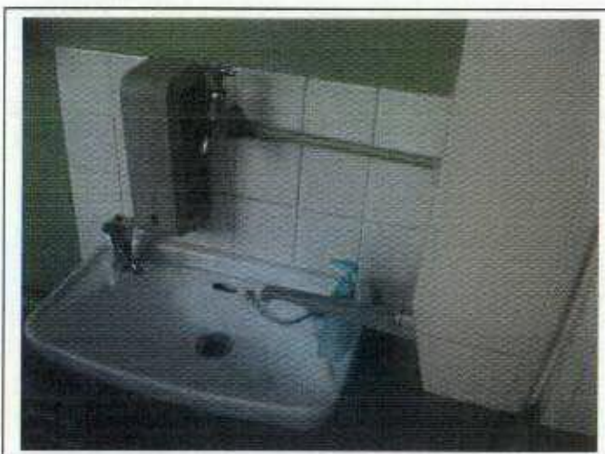
Ground Floor WC 16 Gower Street
