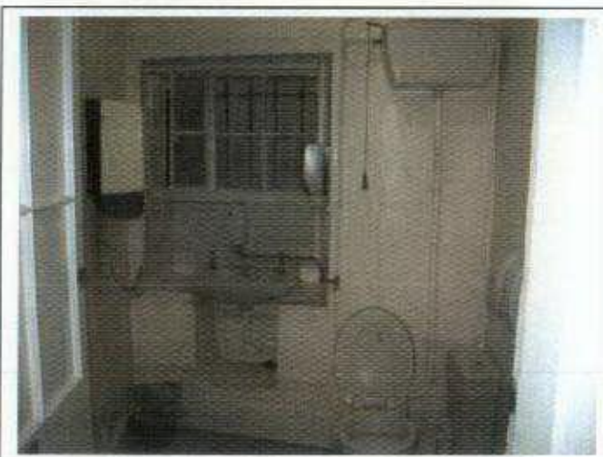
Basement WC 4 Gower Street
