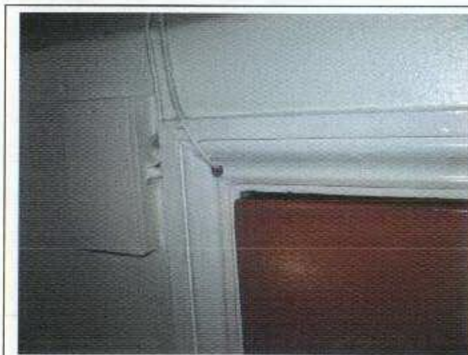
Basement WC 16 Gower Street
