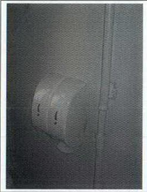
Basement WC 10 Gower Street
