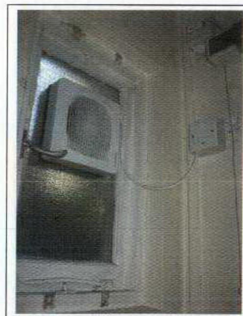
Basement WC 12 Gower Street
