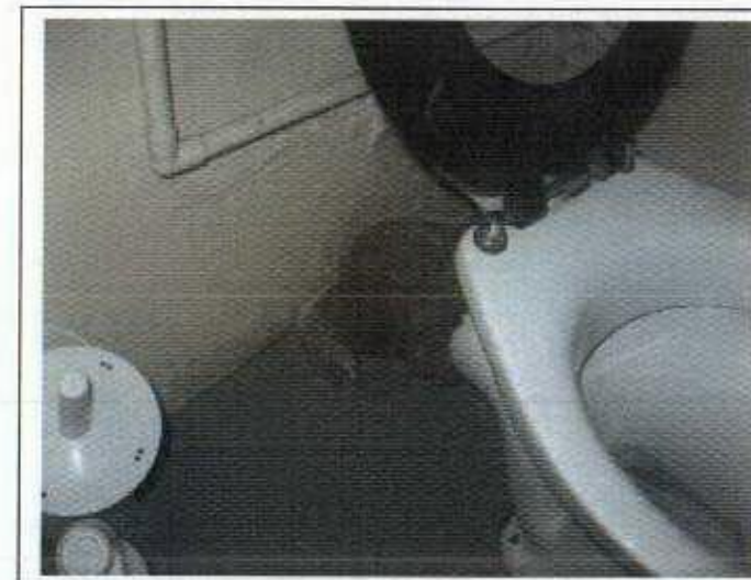
Basement WC 12 Gower Street
