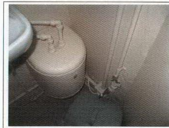
Basement WC 16 Gower Street
