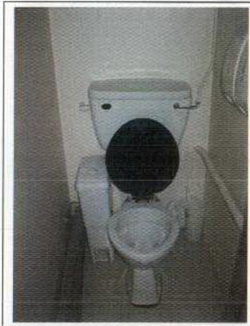
Basement WC 16 Gower Street
