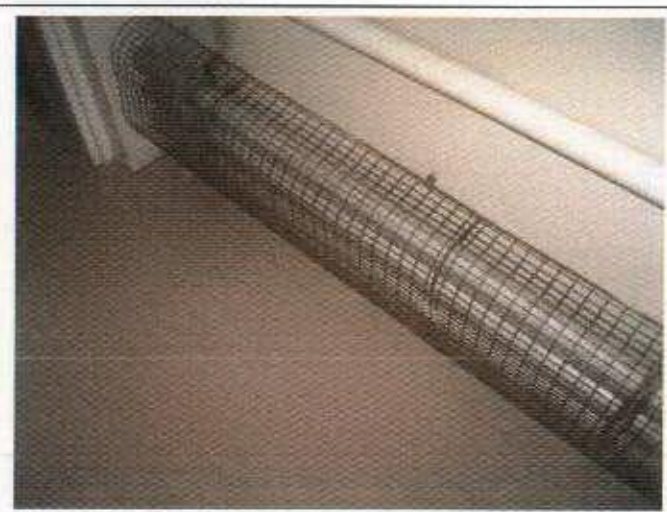
Basement WC 16 Gower Street
