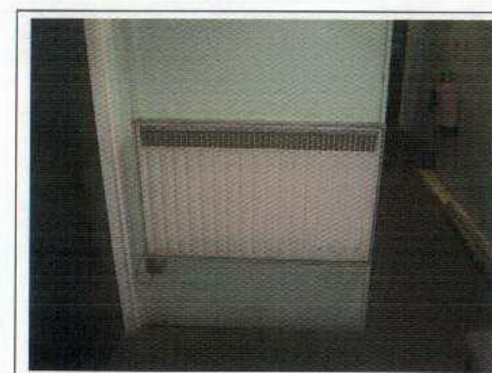
Basement WC 12 Gower Street
