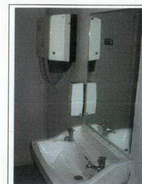
Basement WC 10 Gower Street
