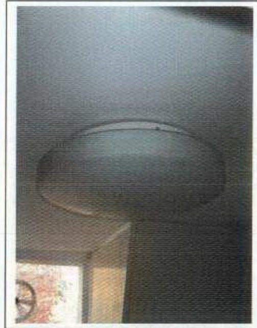
Basement WC 10 Gower Street
