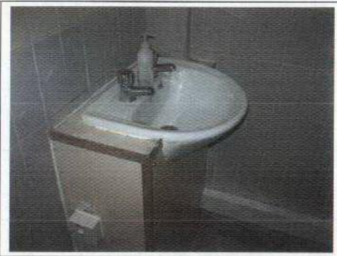
Basement WC's 14 Gower Street
