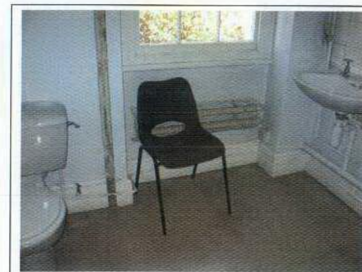
Second Floor WC 12 Gower Street
