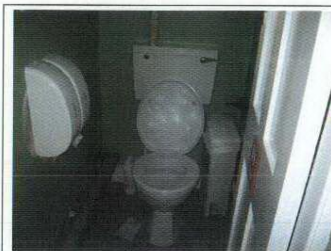
Ground Floor WC 16 Gower Street
