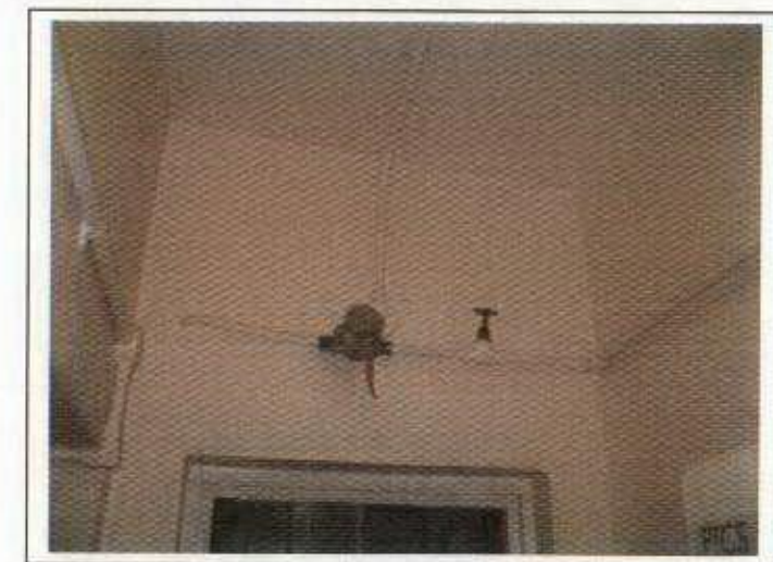
Basement WC 16 Gower Street
