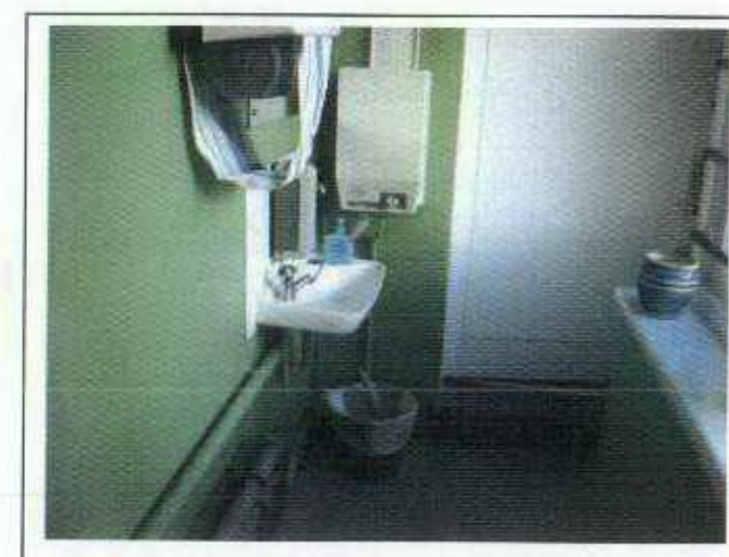
Ground Floor WC 16 Gower Street
