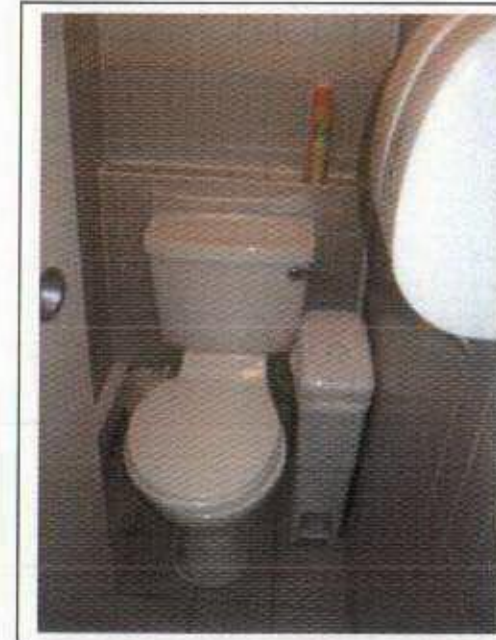
Basement WC's 14 Gower Street
