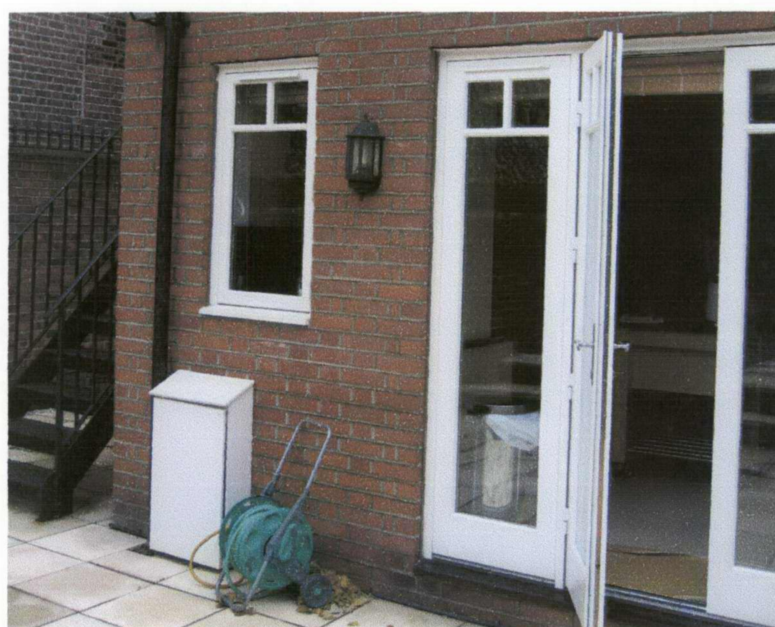
Existing extension- rear facade
