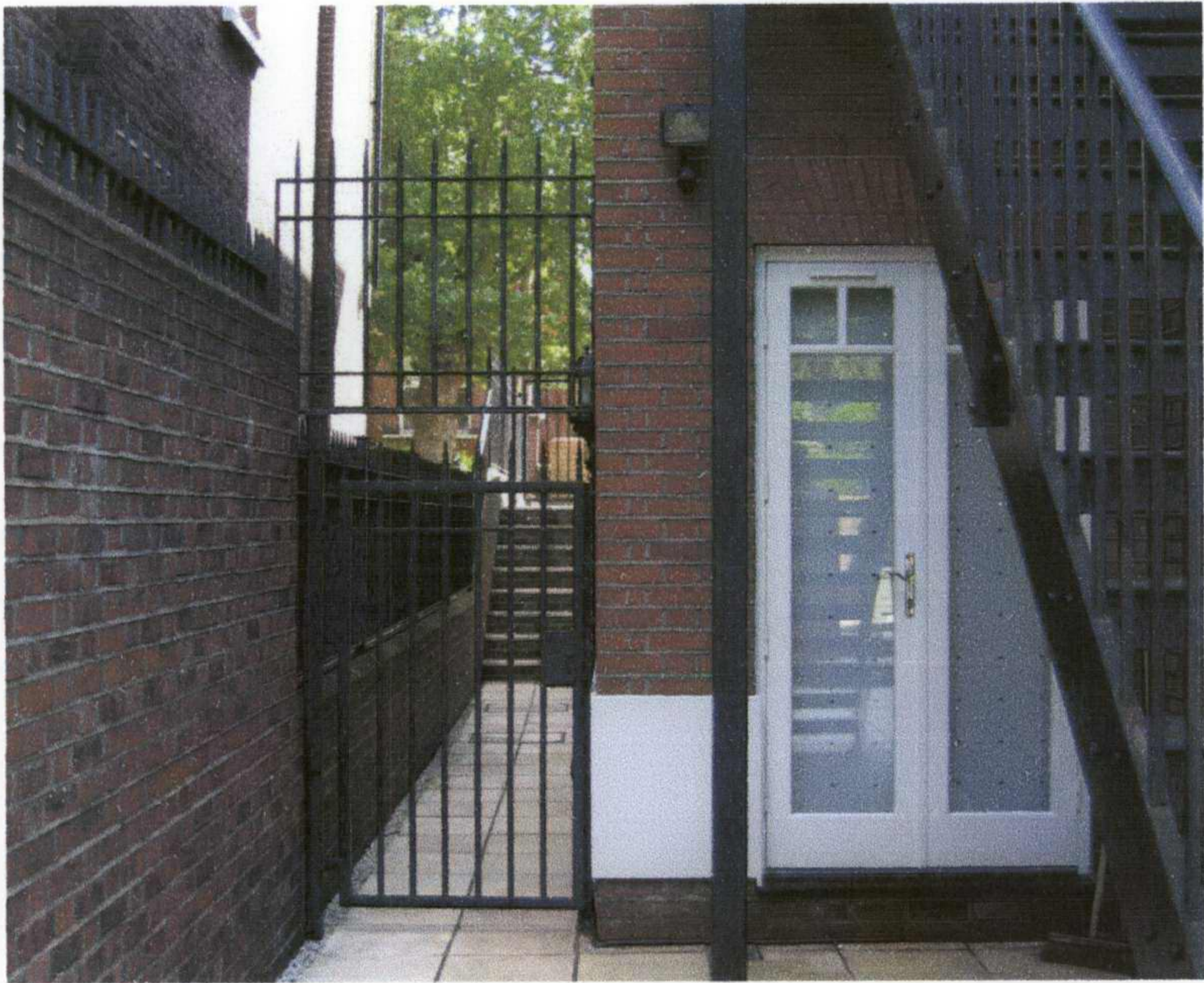
Side passage and detail of Georgian Arch and existing stair
