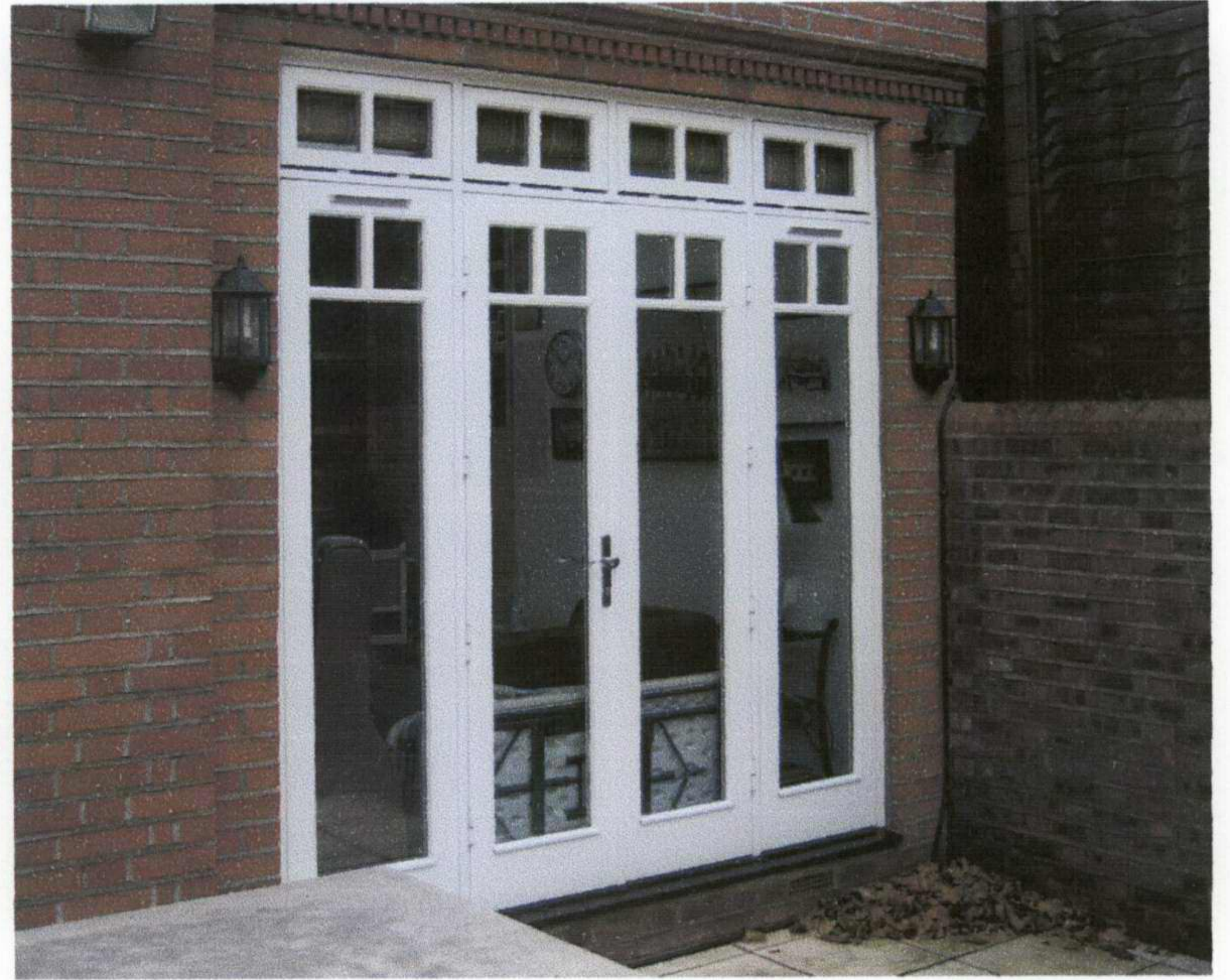
Existing extension. Rear facade
