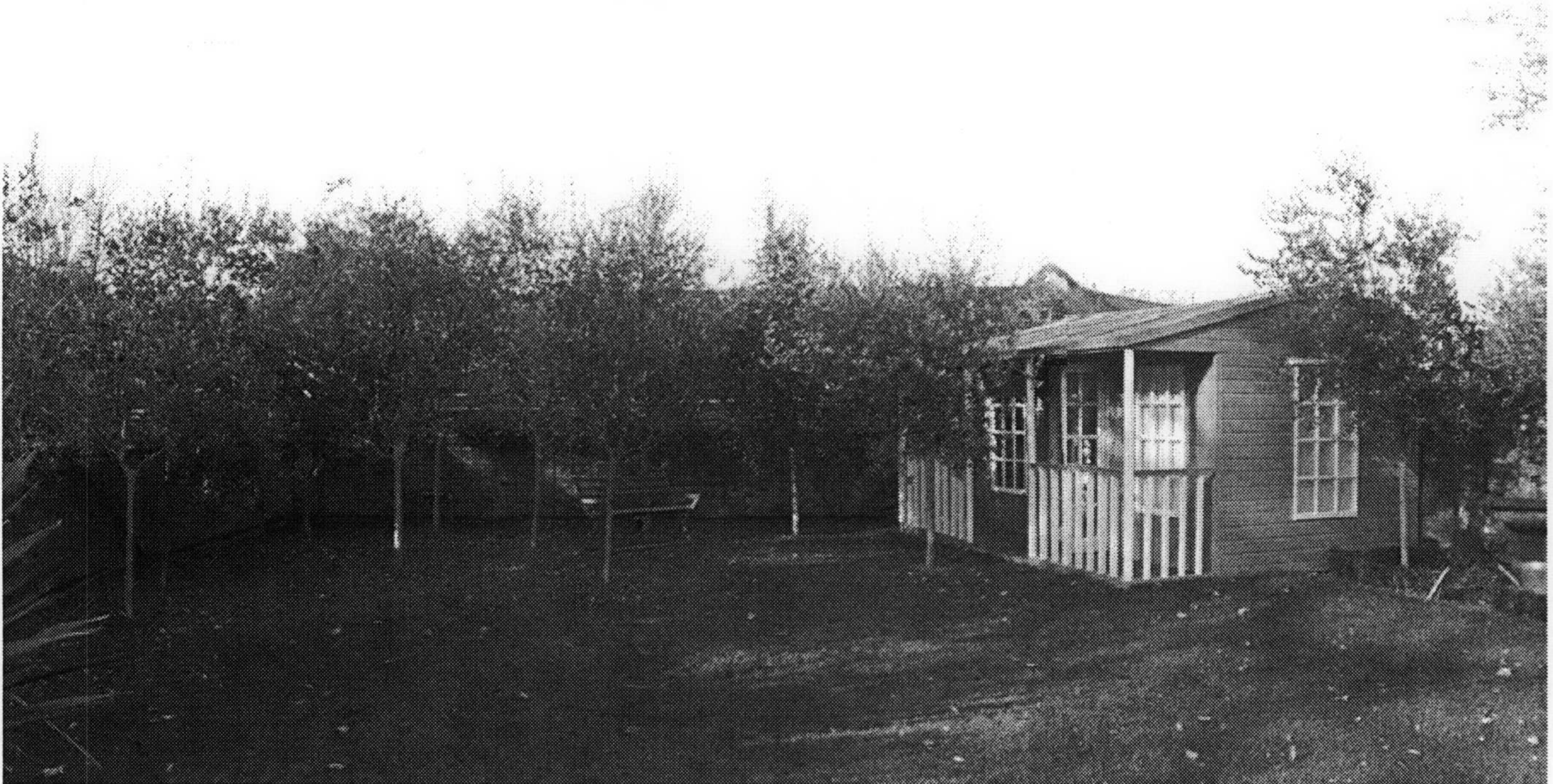
B. View of southwest corner showing relationship to existing olive trees (approximate tree height 4.0 meters)
