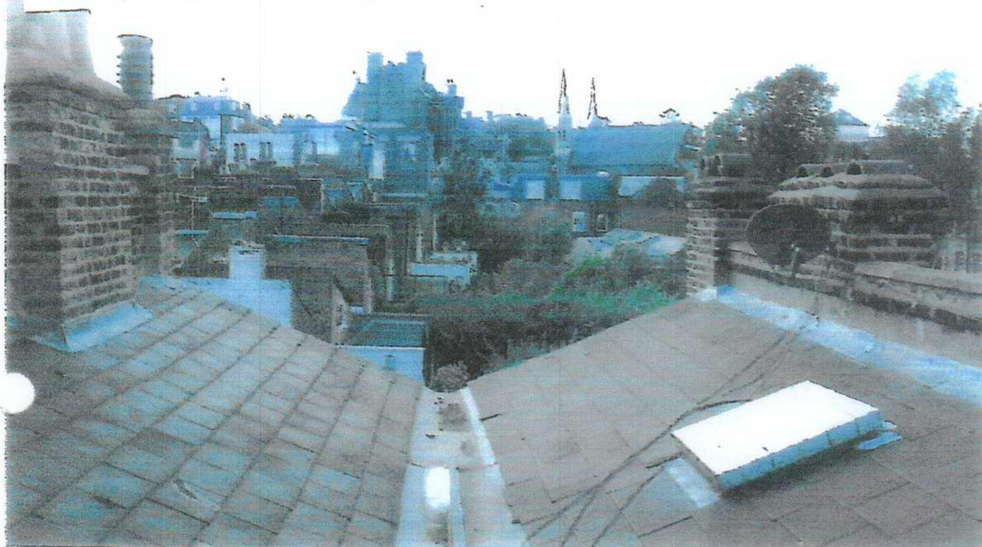
Roof of No. 25
