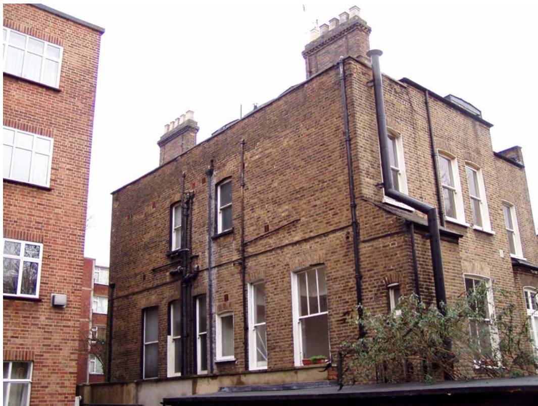
No. 76, showing the various windows and downpipes on the South facade, proposed to be removed and patched, and replaced with a new glazing.
