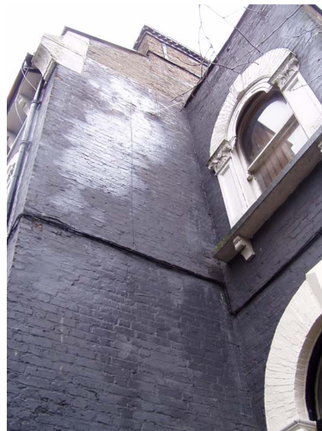
Front facade & entry annex of No. 76, showing the colour paint over the brickwork & bracing to chimney above.
