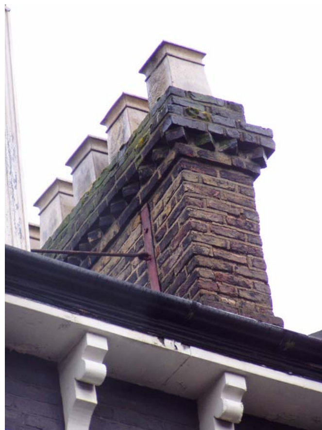
Chimney stack to No. 76, showing the brickwork & bracing to chimney.
