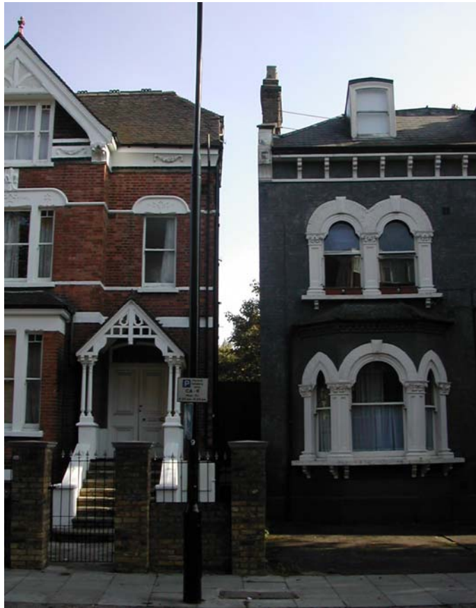
No. 78 (left) & No. 76 (right) Priory Road. View shows the gap between the two buildings, the varying roof forms and the metal rods bracing the chimney stacks to the roof.
