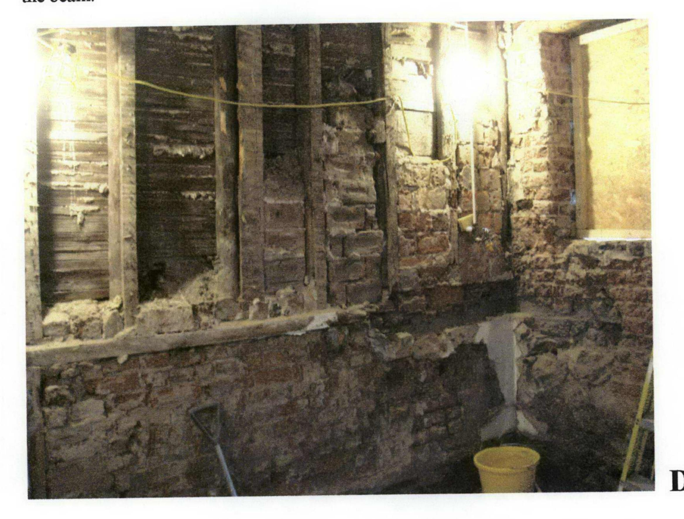
A broader view of the corner of the stair wall from the room side. Outside the far corner is the drain which caused the damage to the fabric.
