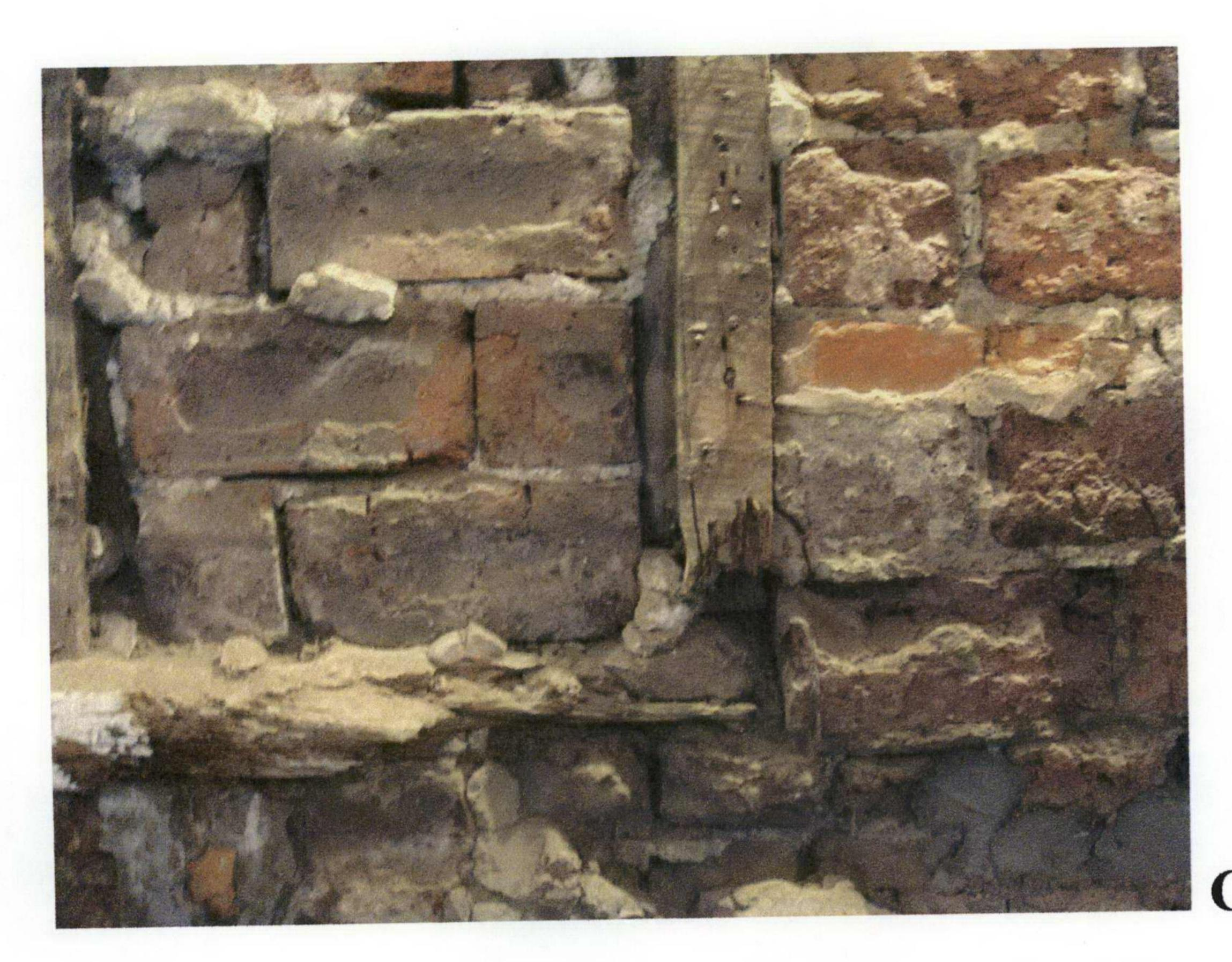
Timber within the wall is rotting, while masonry is only fill, not capable of offering support to the beam.
