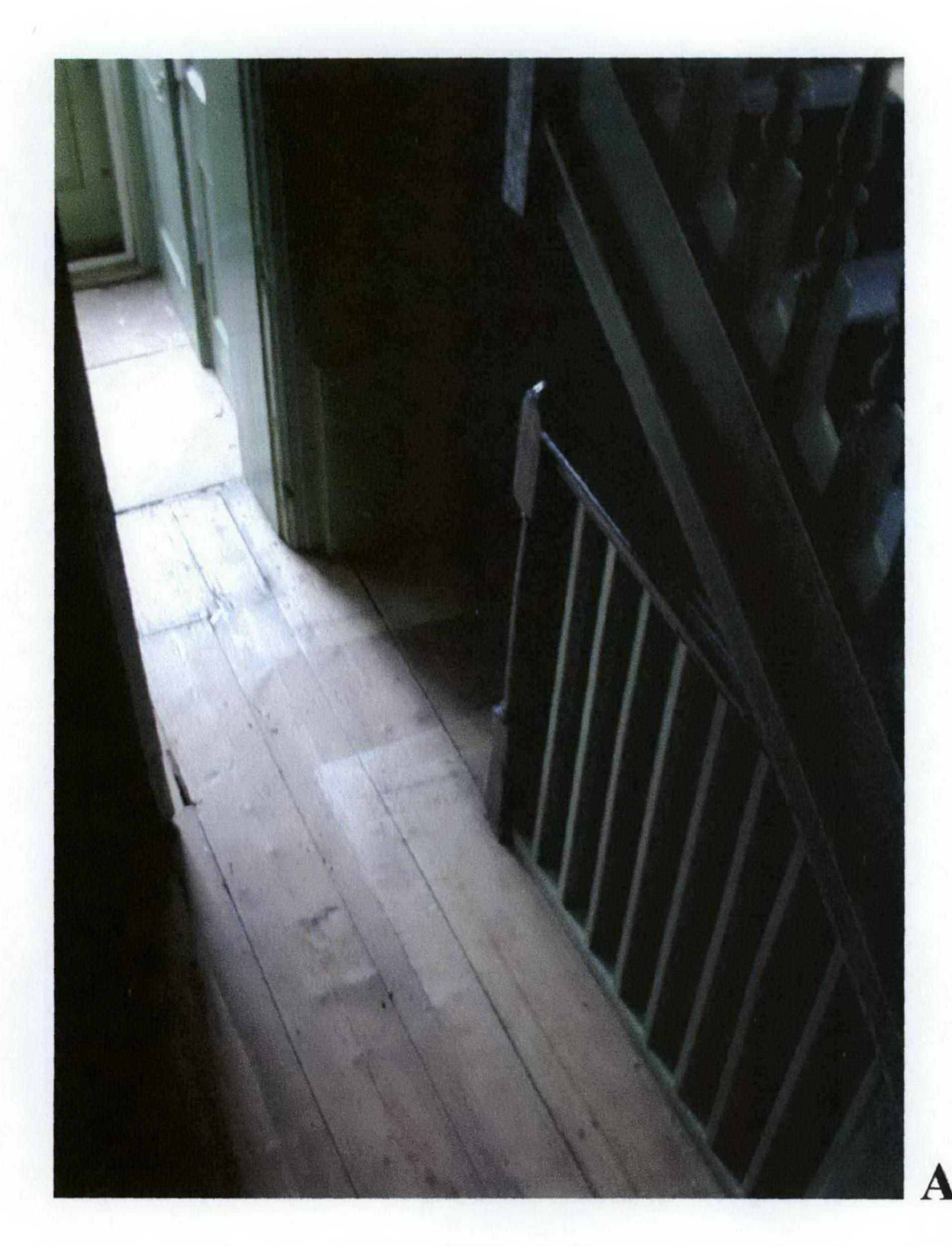
Photograph showing the top of the stair from the ground floor hall. The Dark line from the post to the back wall would be the first step down in the proposed new arrangement.
