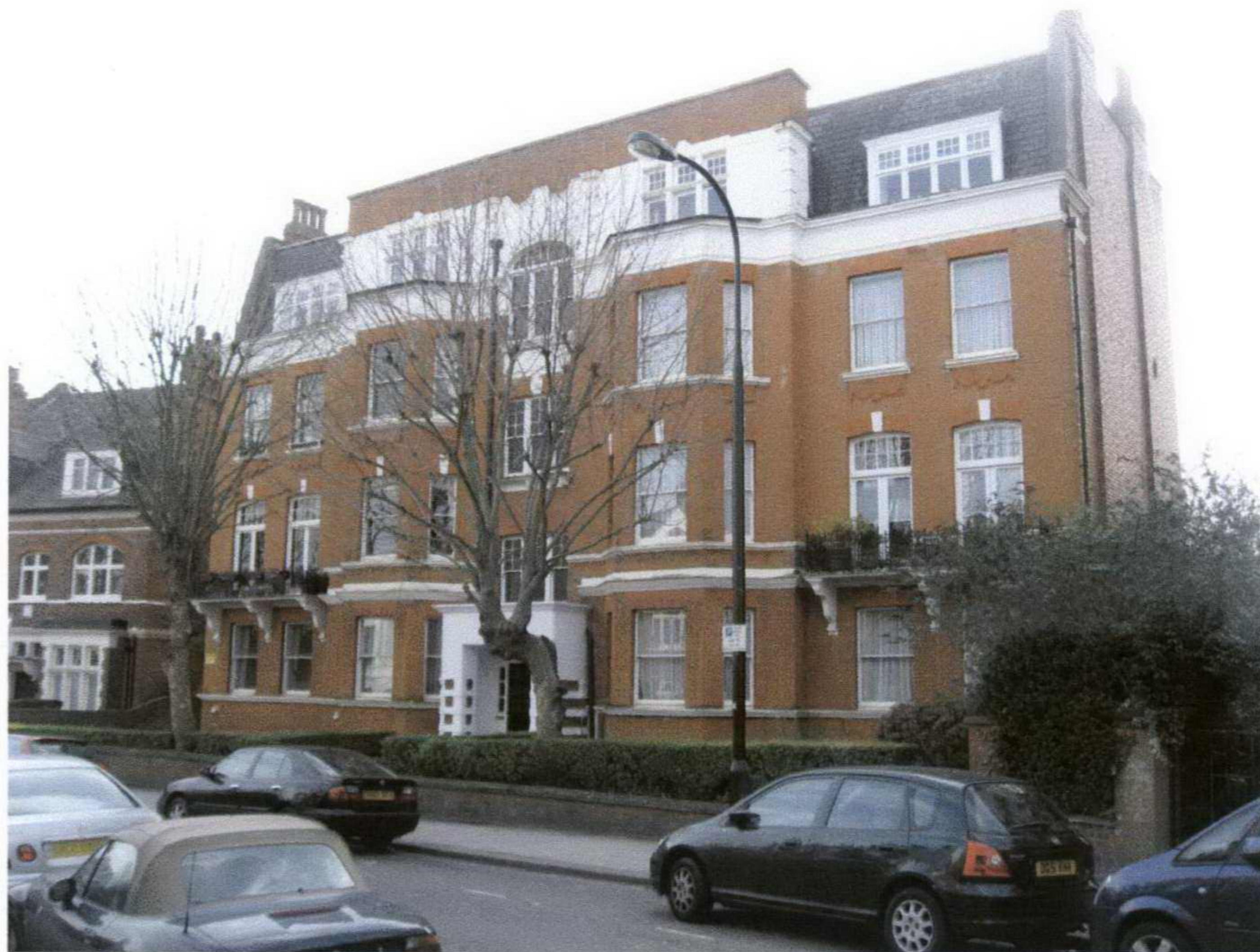
125-139 BROADHURST GARDENS - FRONT VIEW
