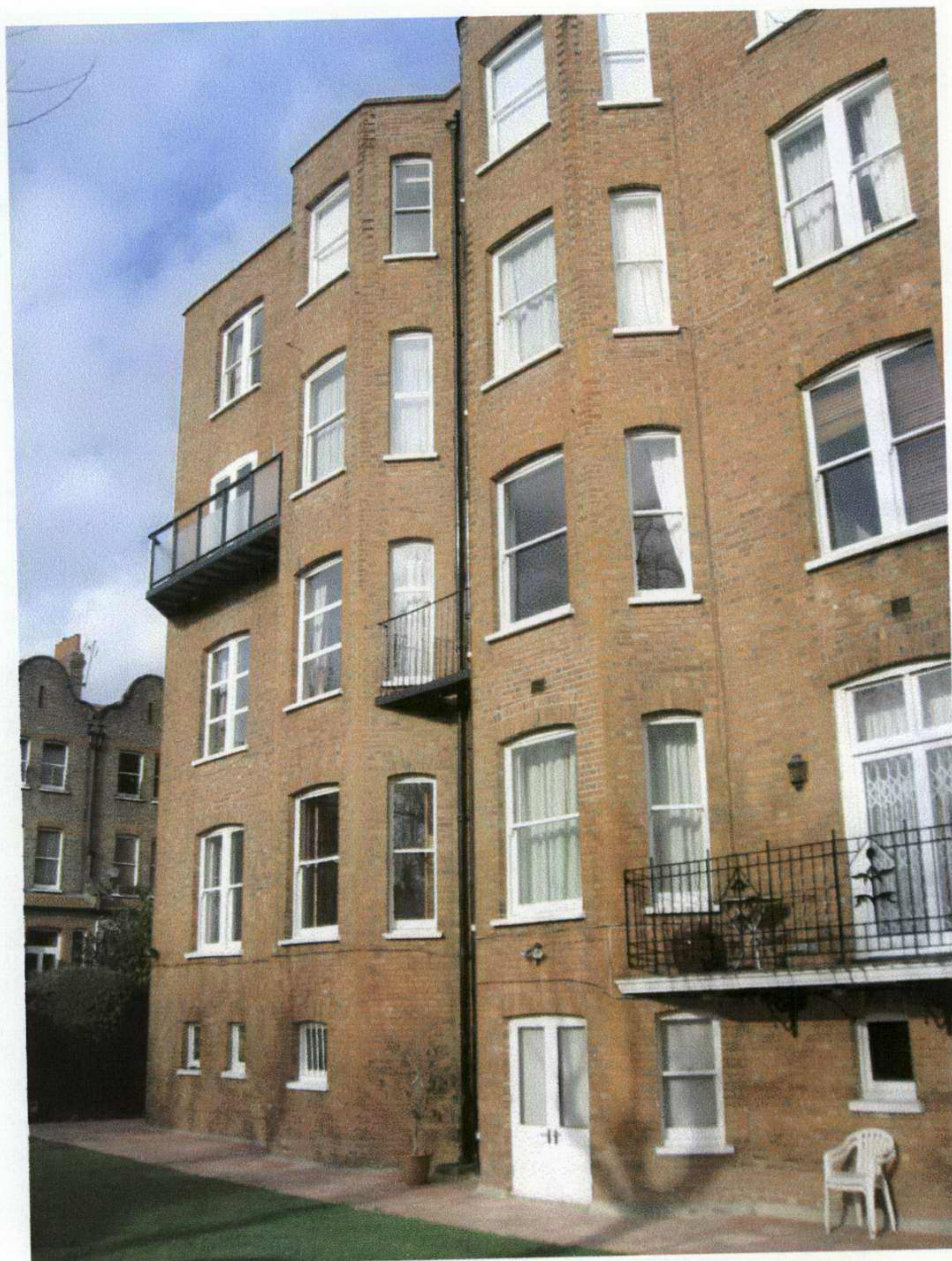
REAR OF BLOCK FROM COMMUNAL GARDEN, LOOKING N.W.
