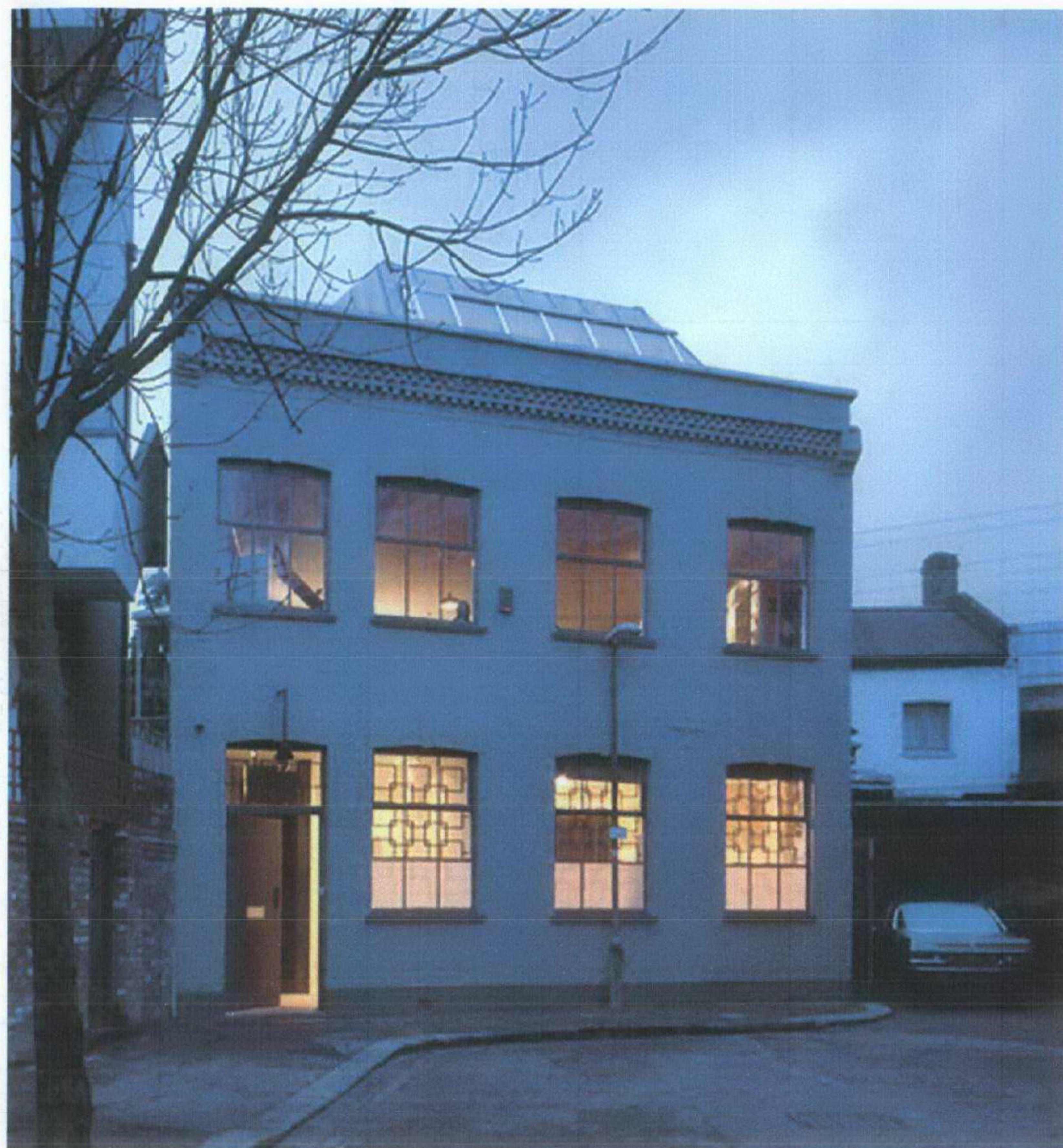
Phase 1 as completed, showing the Terne Coated Steel mansard roof (B) and in-line rooflights (F)
