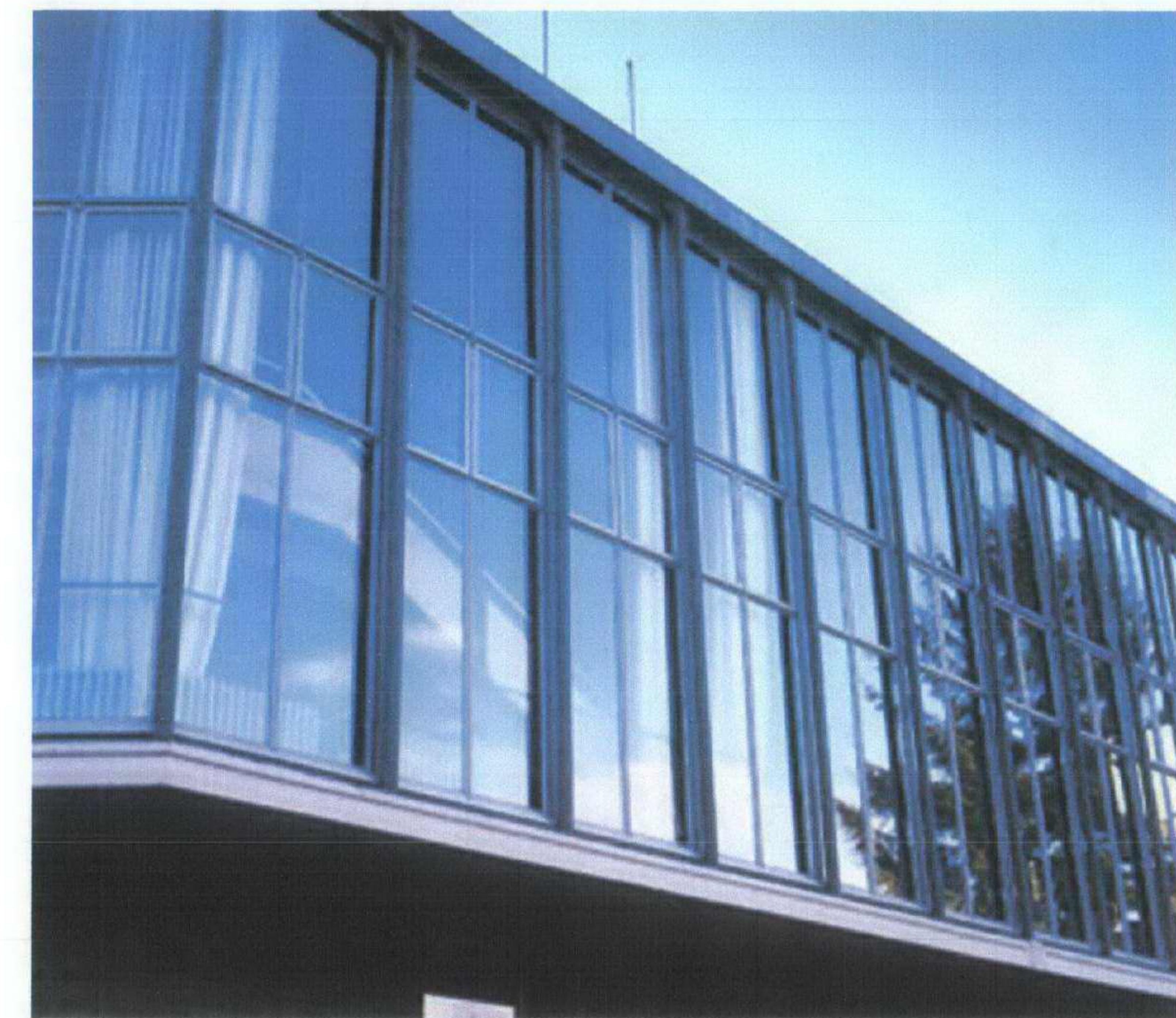
(G) Steel framed Crittall type windows
