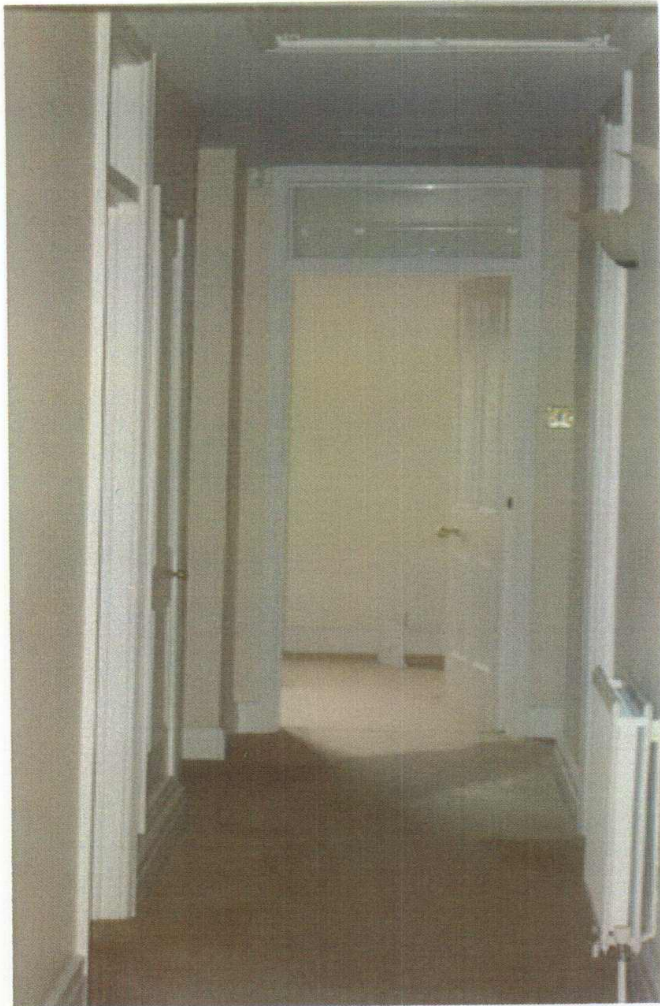
Plate 1: Door to be blocked up
