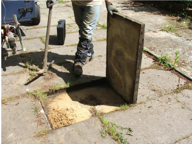
Plate 3: (photo 3385) showing lifted paving in relation to T6
