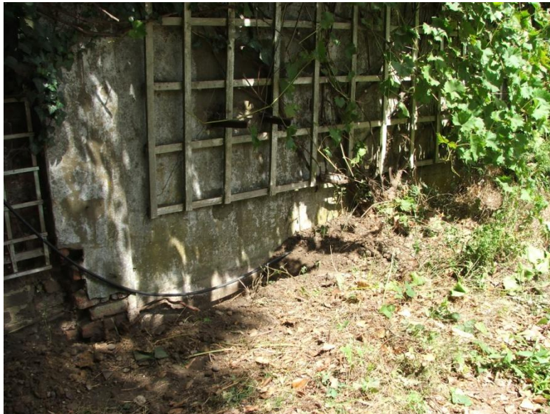
Plate 4: (photo 3376) showing excavated trench in relation to T7
