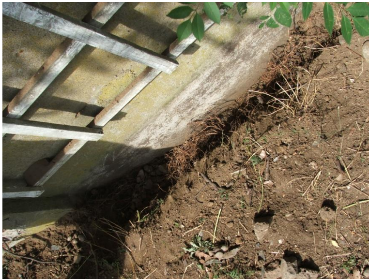
Plate 2: (photo 3383) showing excavated trench in relation to T6
