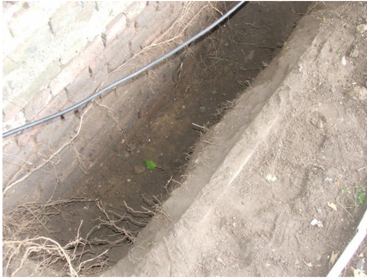
Plate 5: (photo 3367) showing excavated trench in relation to T10
