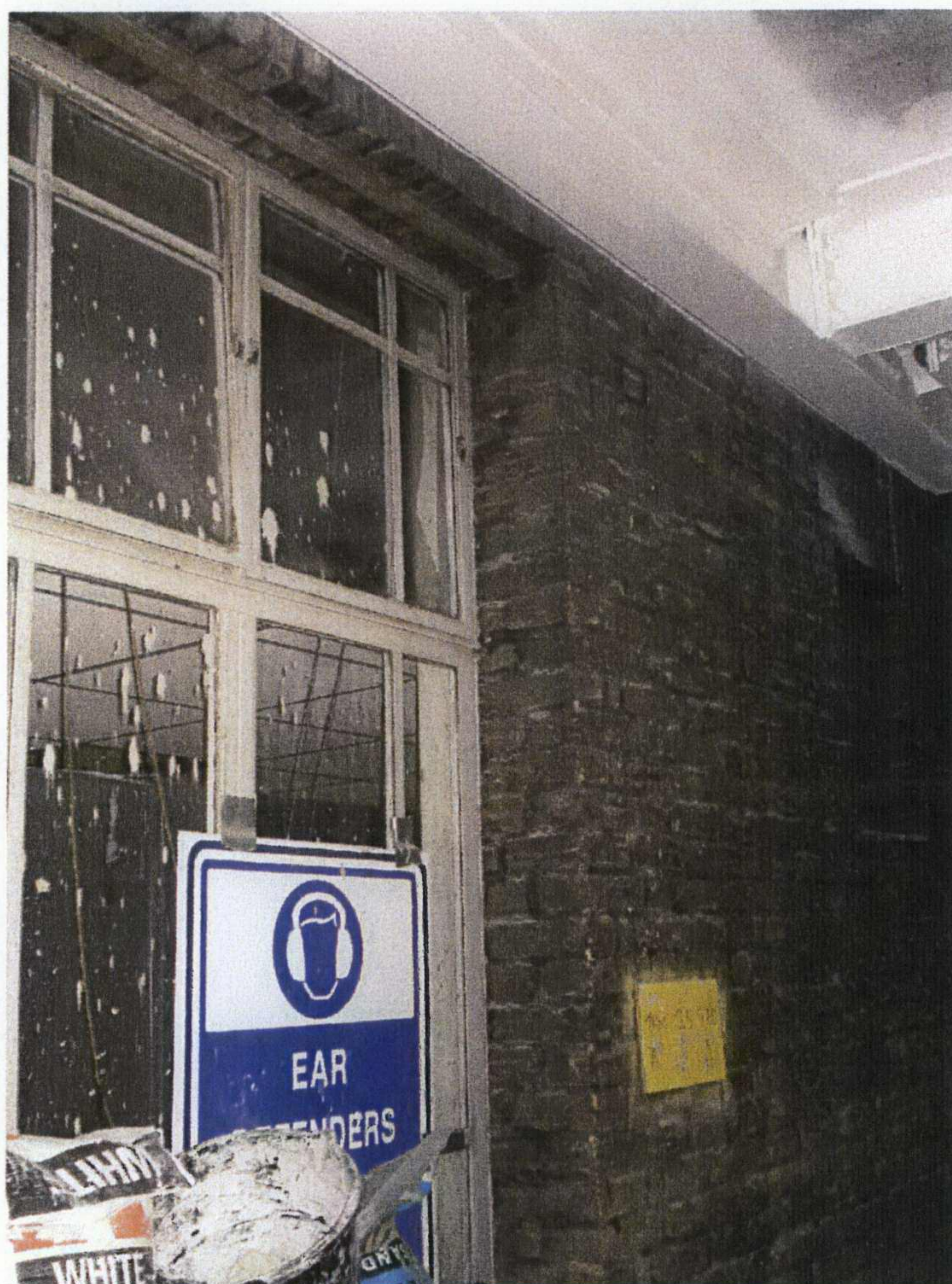
5. Lobby Area – Dry Riser penetration, Internal window W/LG/W/04 (North).
