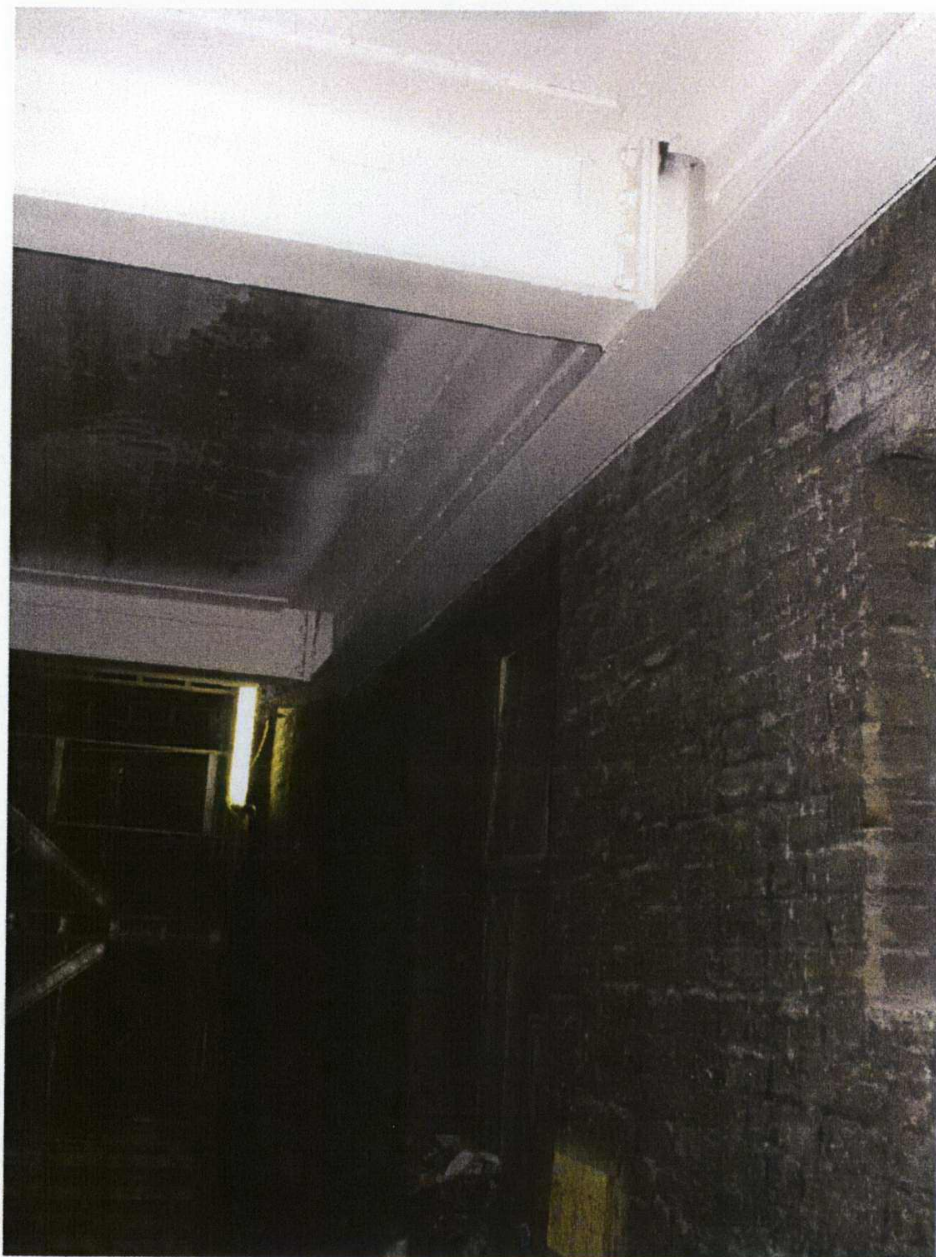
3. Lobby Area – Dry Riser penetration, Internal window W/LG/VV/04 (South).
