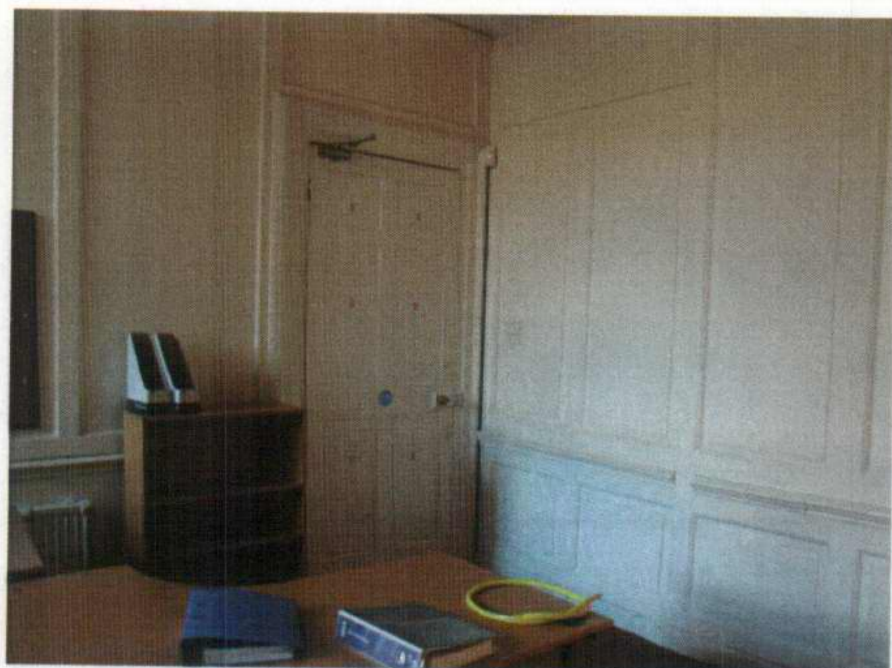
Figure 41 Room F19. Where overpanelling occurs, panels to be carefully removed to see if any original panelling remains below.
