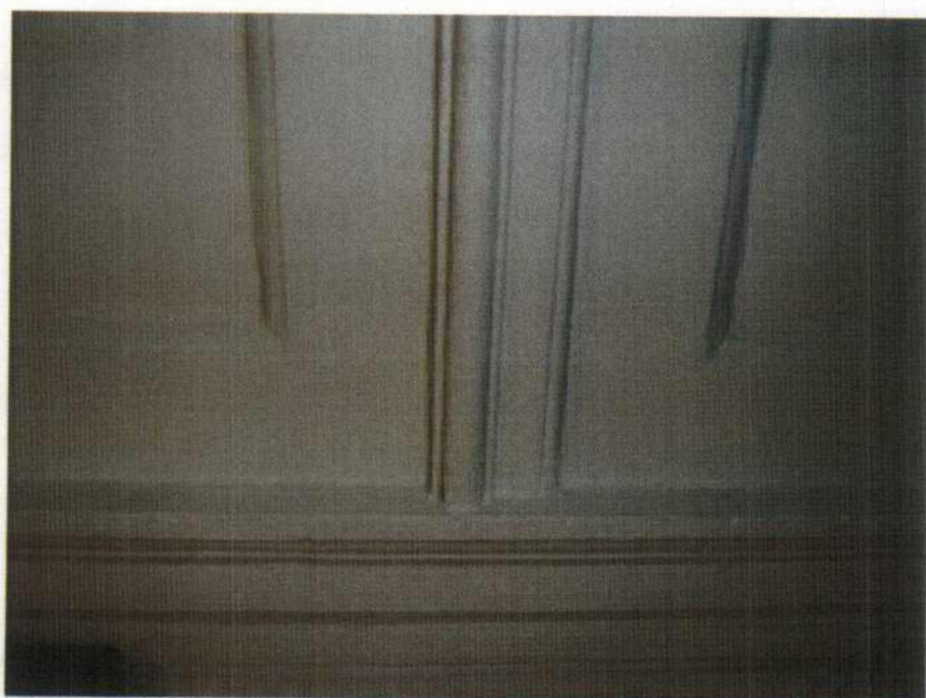
Figure 35 Detail of panel and dado
