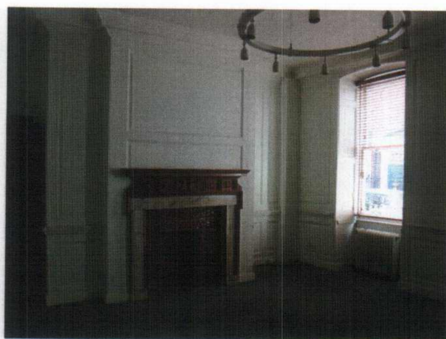
Figure 36 Room B6, duct to corner to be removed, modern tiled insert to fire surround to be replaced with appropriate insert.
