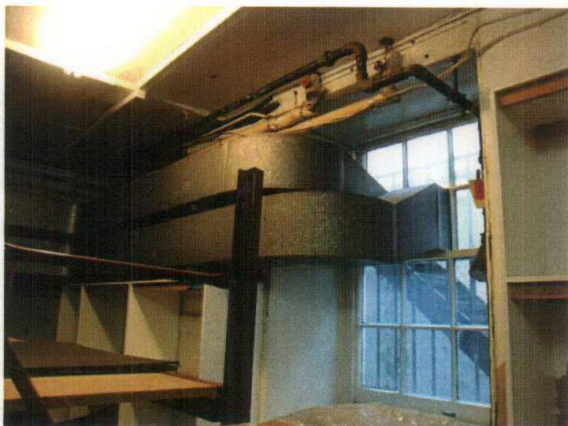
Figure 25 Room B4, extensive ducting to be removed and windows overhauled and glazing reinstated.
