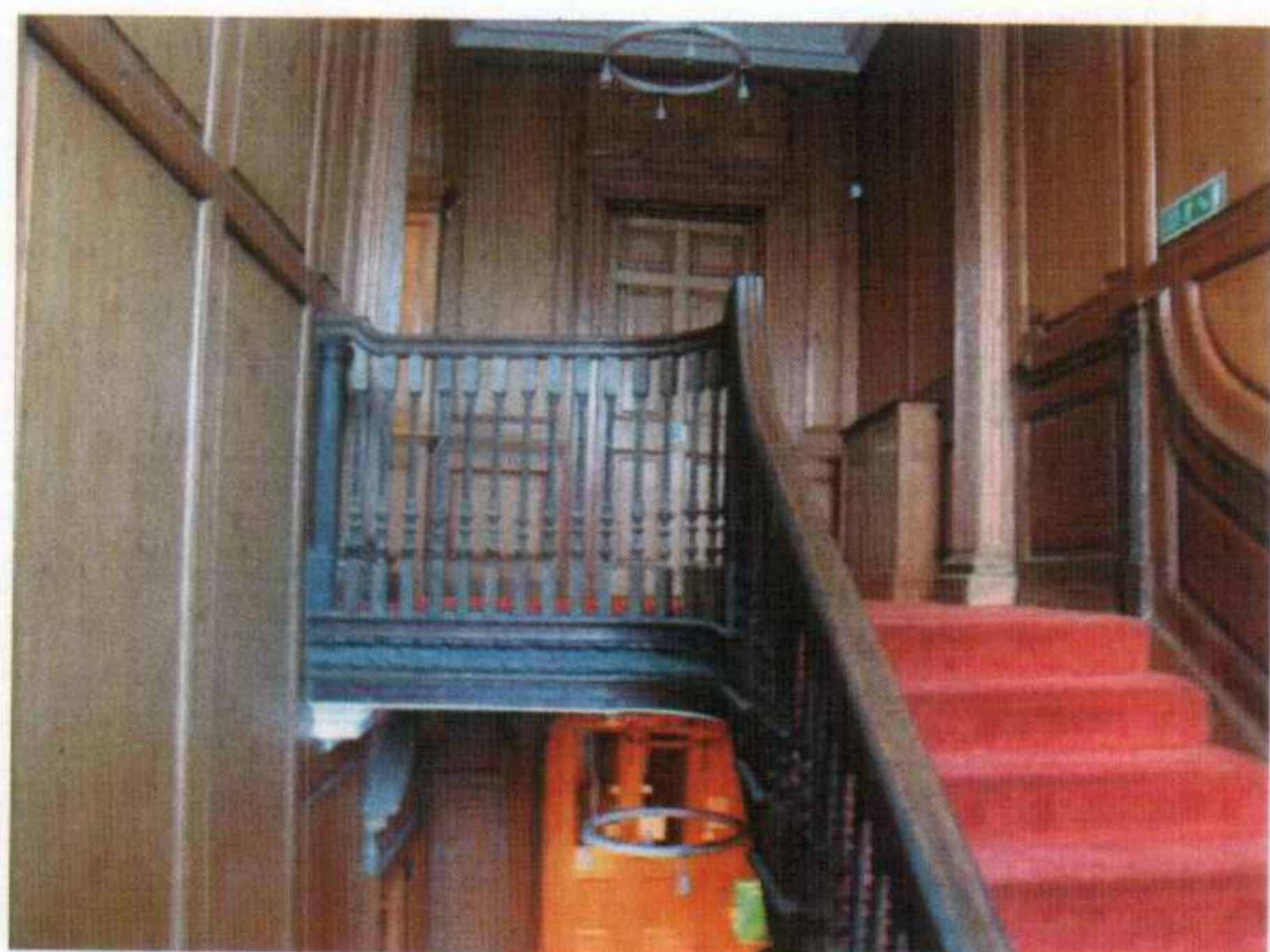
Figure 39 Polished oak balustrade, handrail and below dado panelling to stair to no. 12. Stripped panelling above dado to be re-painted.
