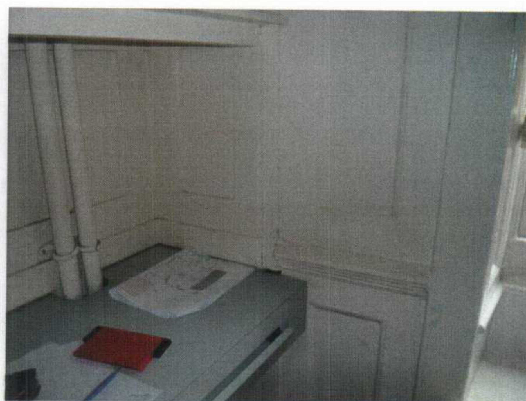
Figure 34 Simple panelling in recesses. Cupboard doors to be reinstated.
