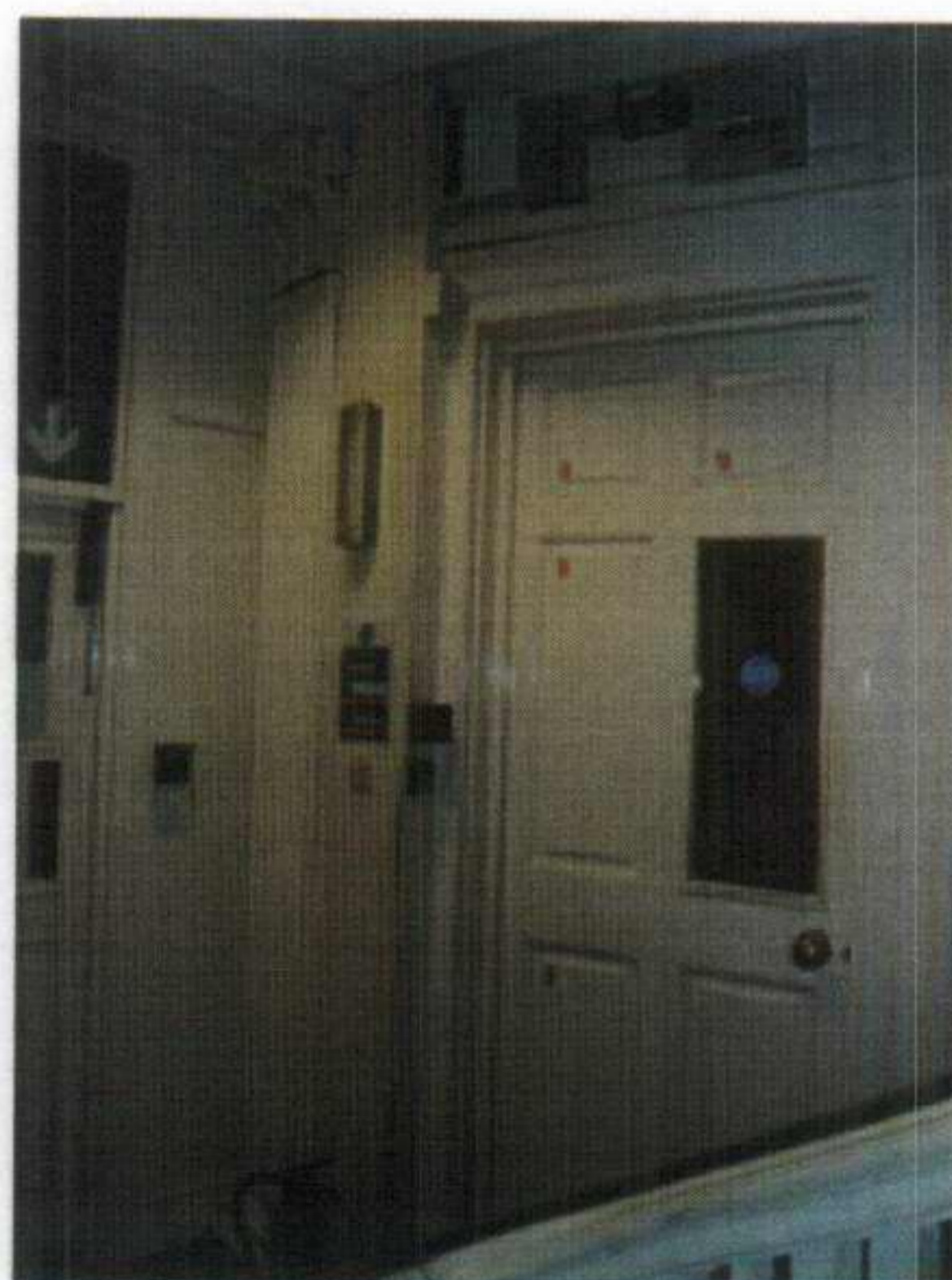
Figure 28 Riser in stair to no. 11 to remain. Glazed panel in door to be reinstated as solid panel.
