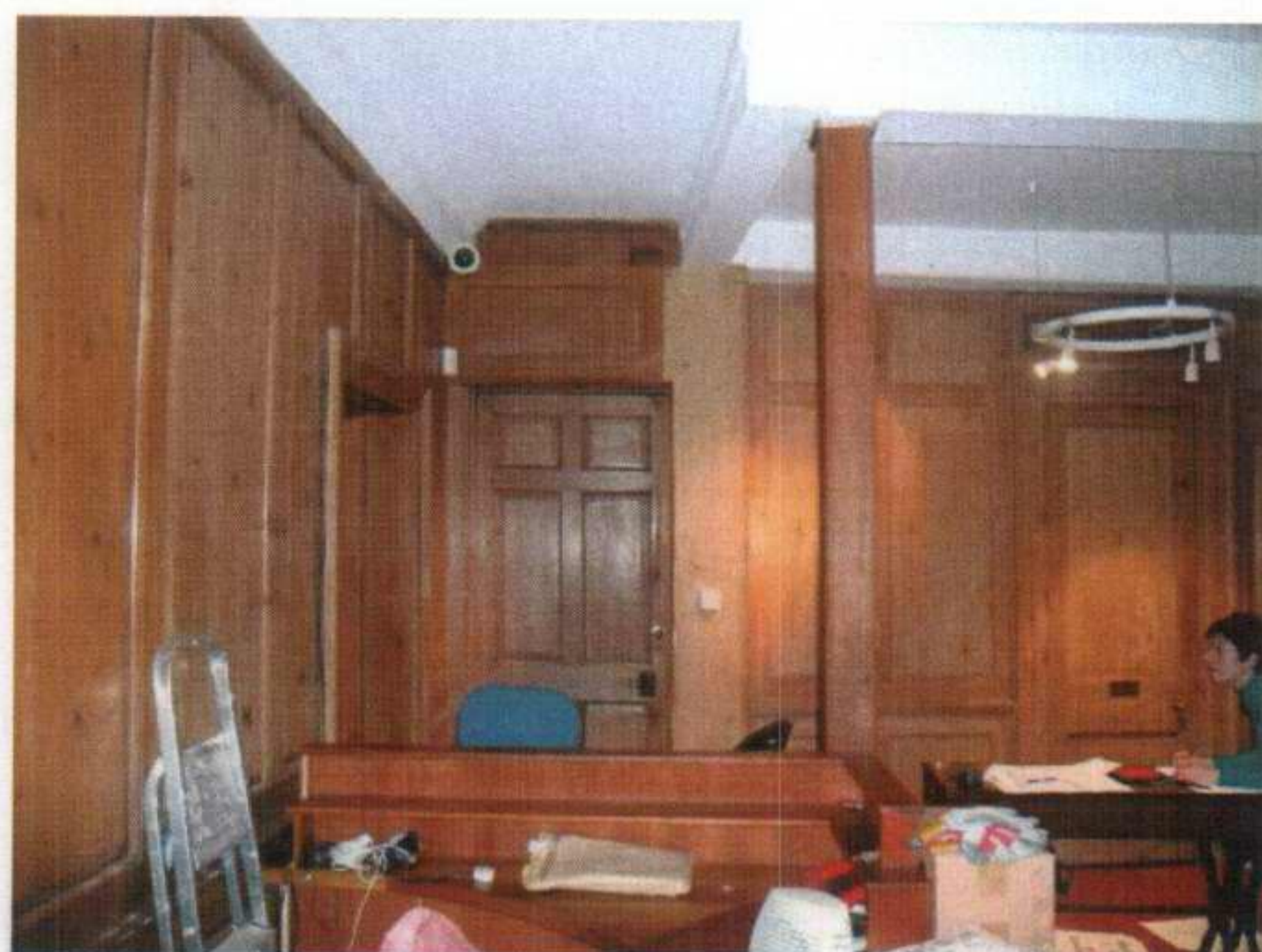
Figure 22 Stripped panelling to G6. Column to be removed and new beam inserted. Panelling to be re-painted.
