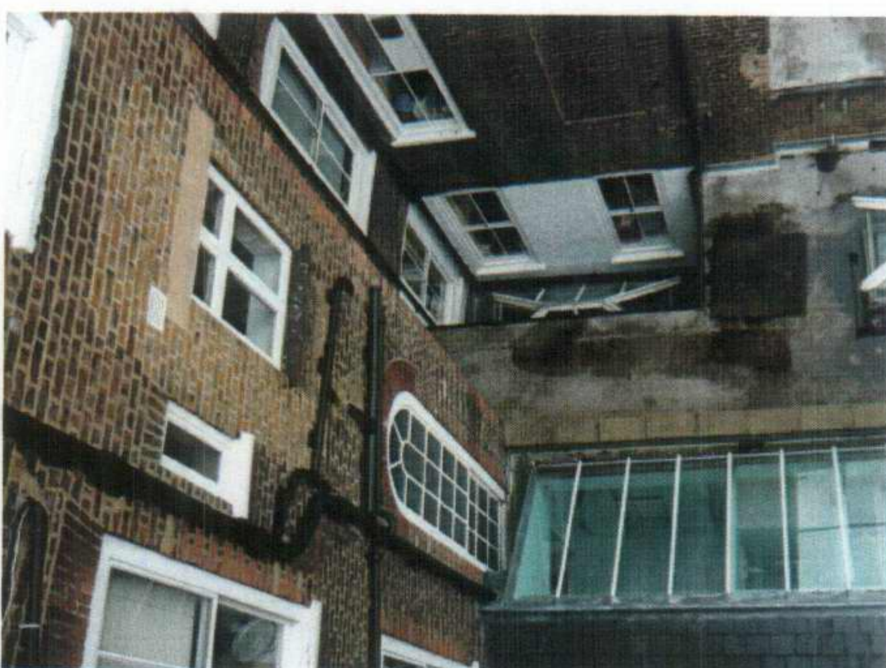
Figure 5 Rear Elevation to no.12. showing alterations to windows. Original window configuration to be reinstated.
