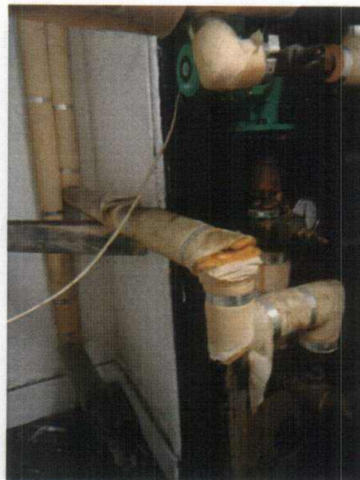
Figure 20 Room B3, pipework around existing range to be removed and range refurbished and exposed.
