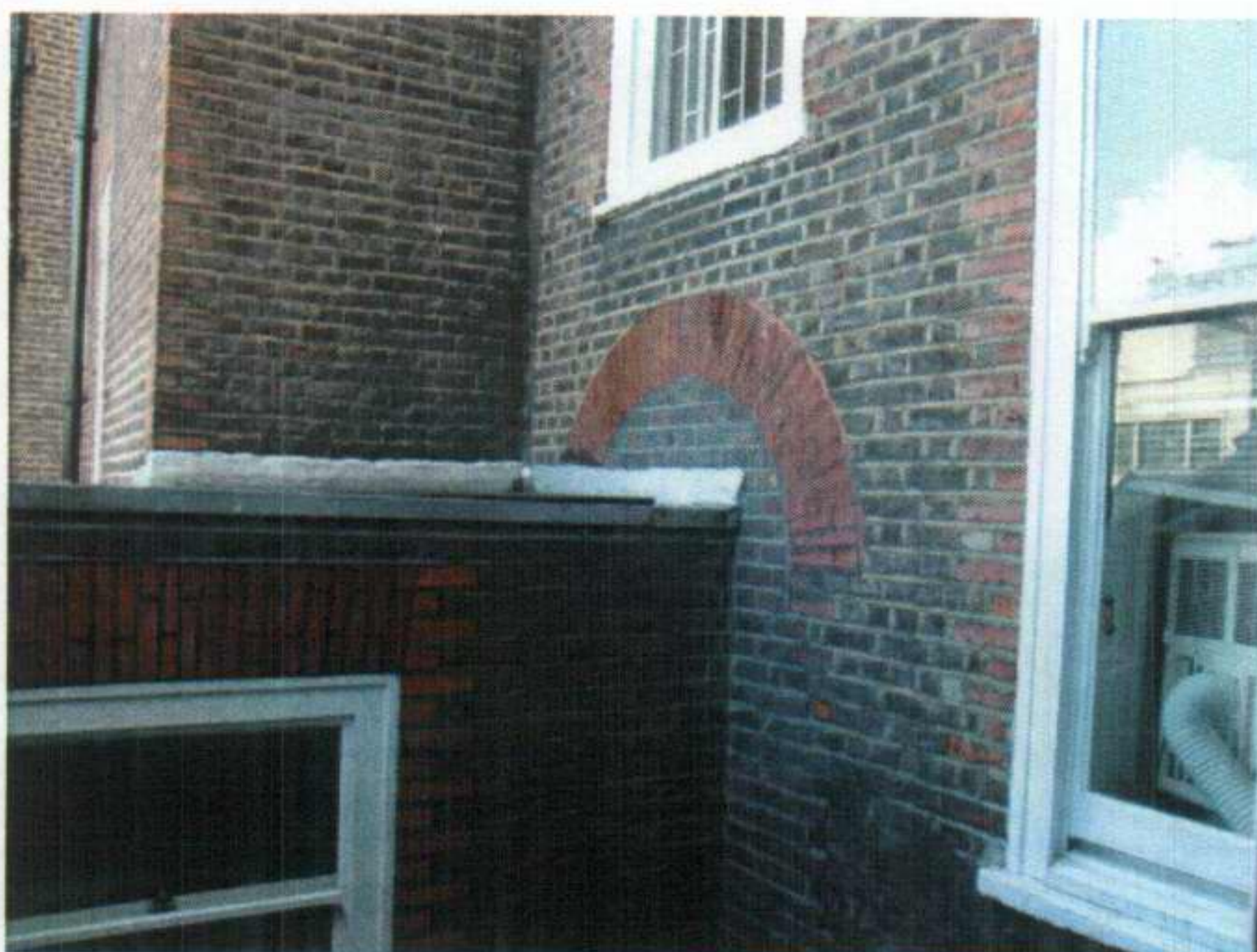
Figure 3 No 11, modern two storey extension, external junction with historic house. Original arched window to stair to be reinstated
