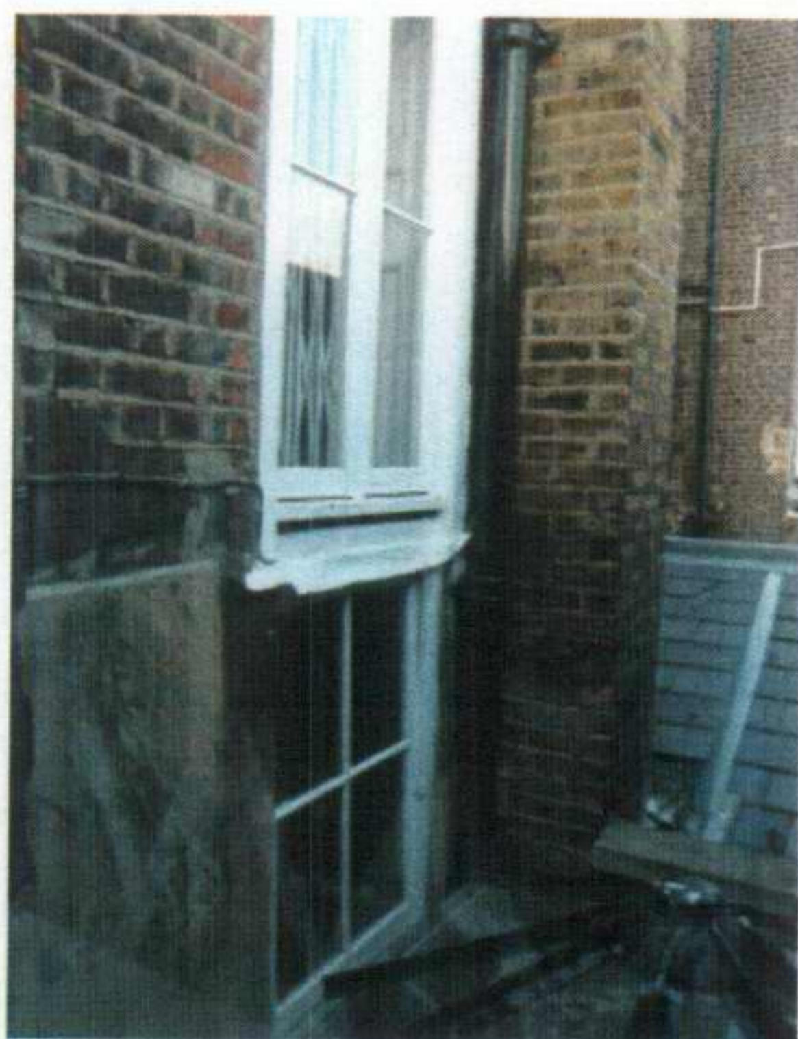
Figure 11 Window alterations to rear of no.12. Low level window to remain, new sash window to upper level. Render to be carefully removed
