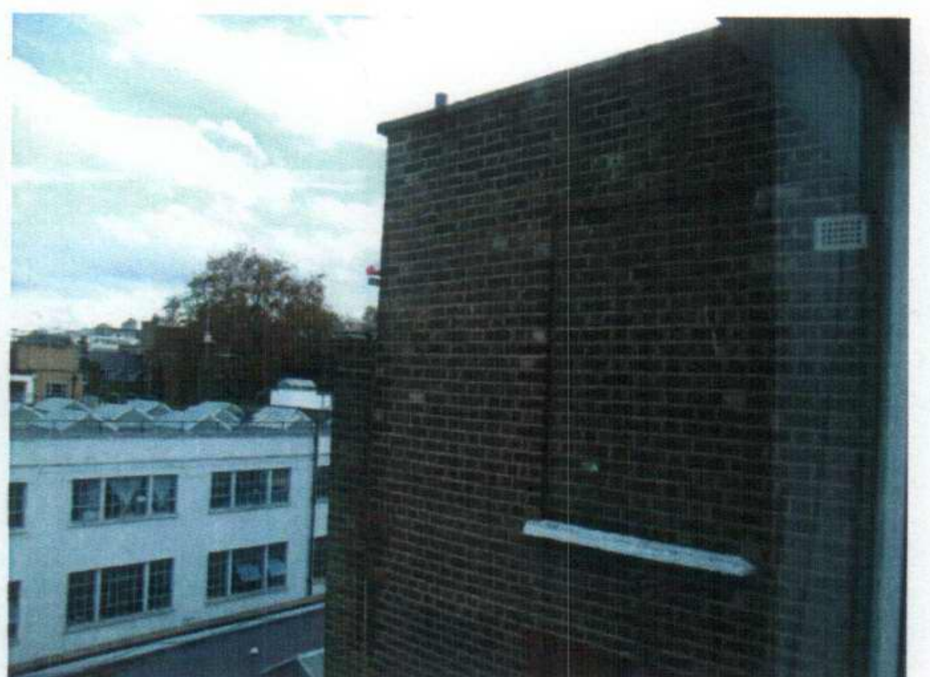
Figure 6 Third floor annexe probably re-built post war with added buttress.
