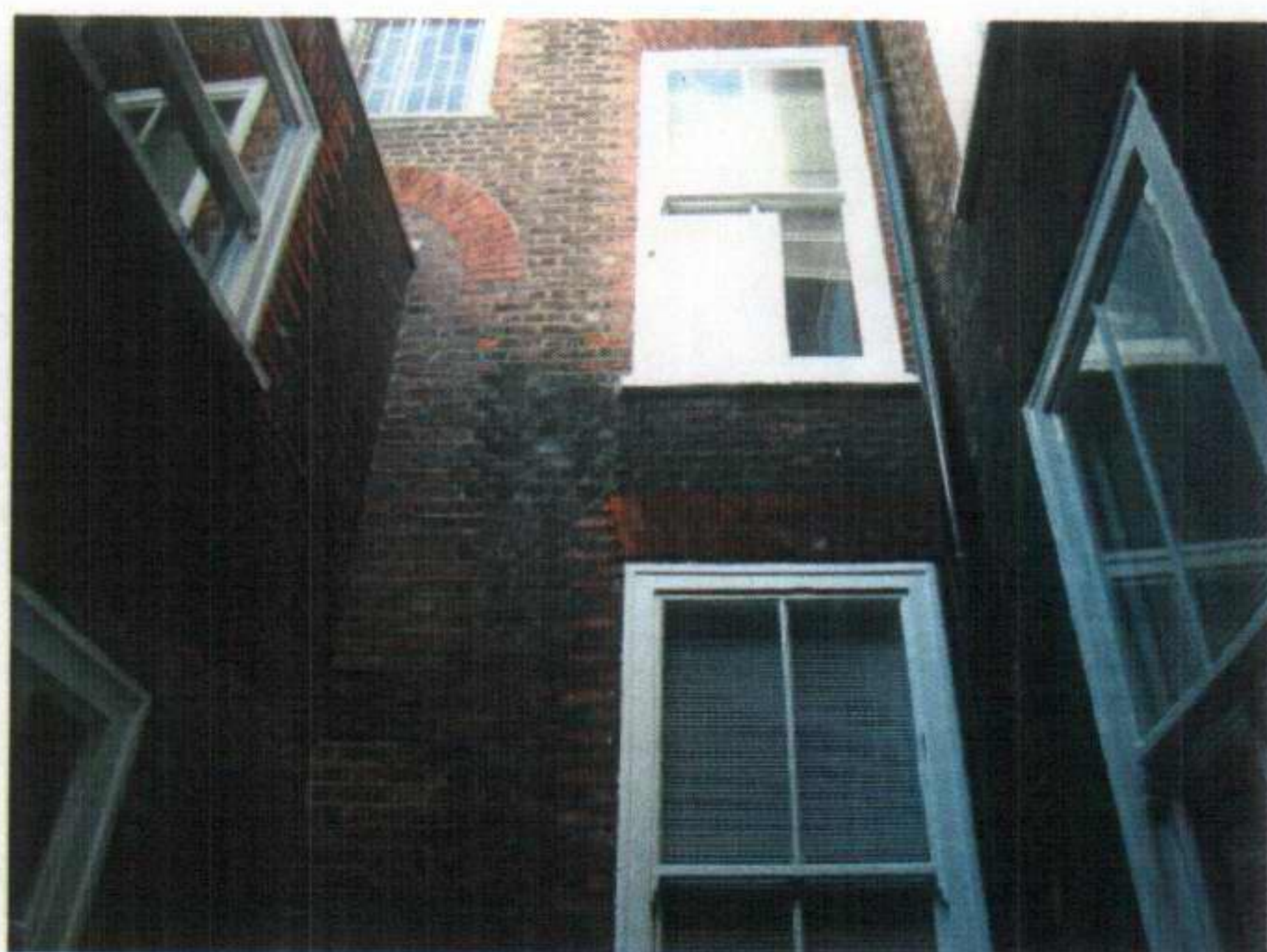
Figure 23 View of existing two storey extension and existing lightwell to no. 11. Original bricked up window locations also visible.
