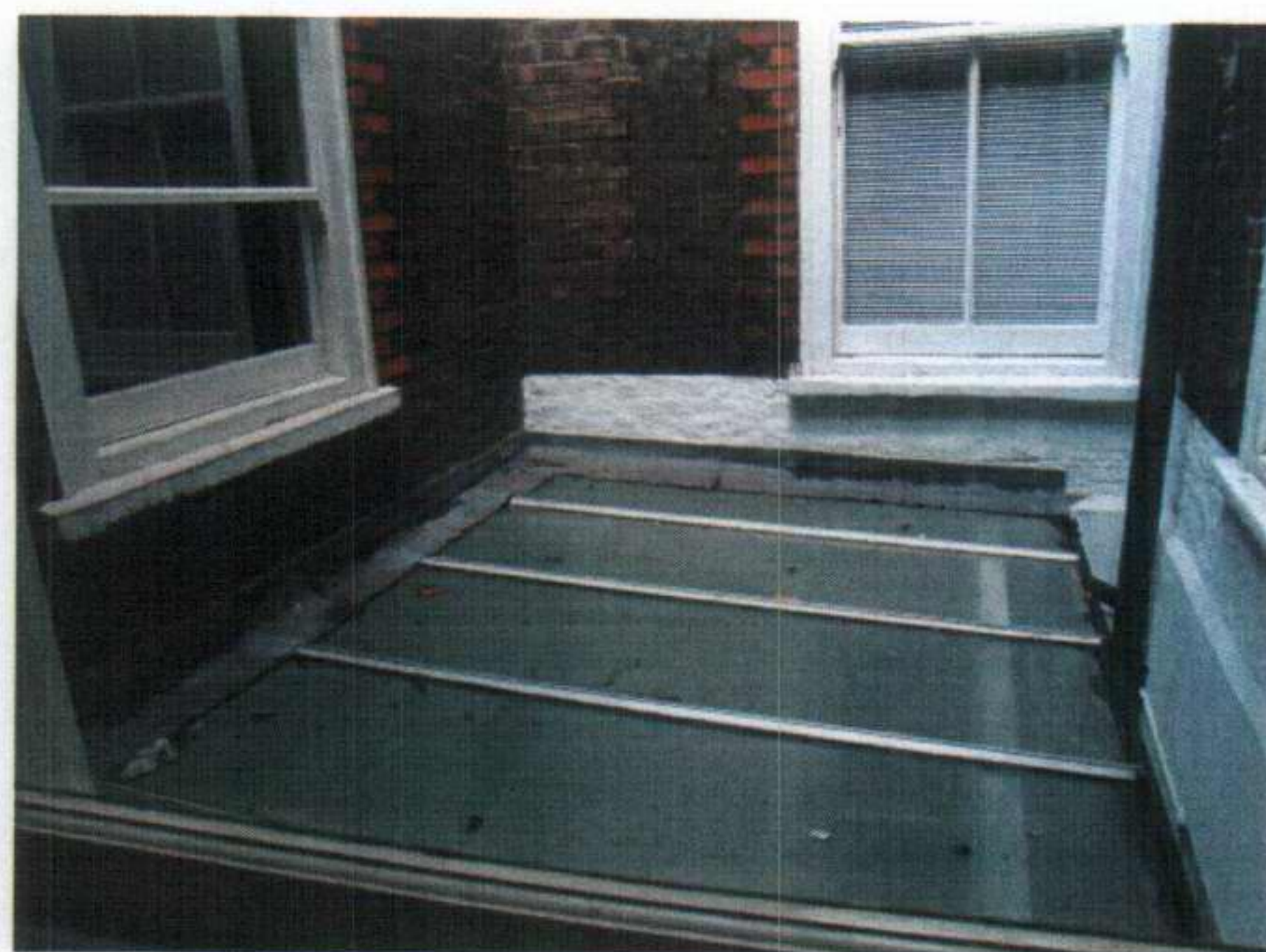
Figure 14 Remove glazed roof to existing lightwell to no.11
