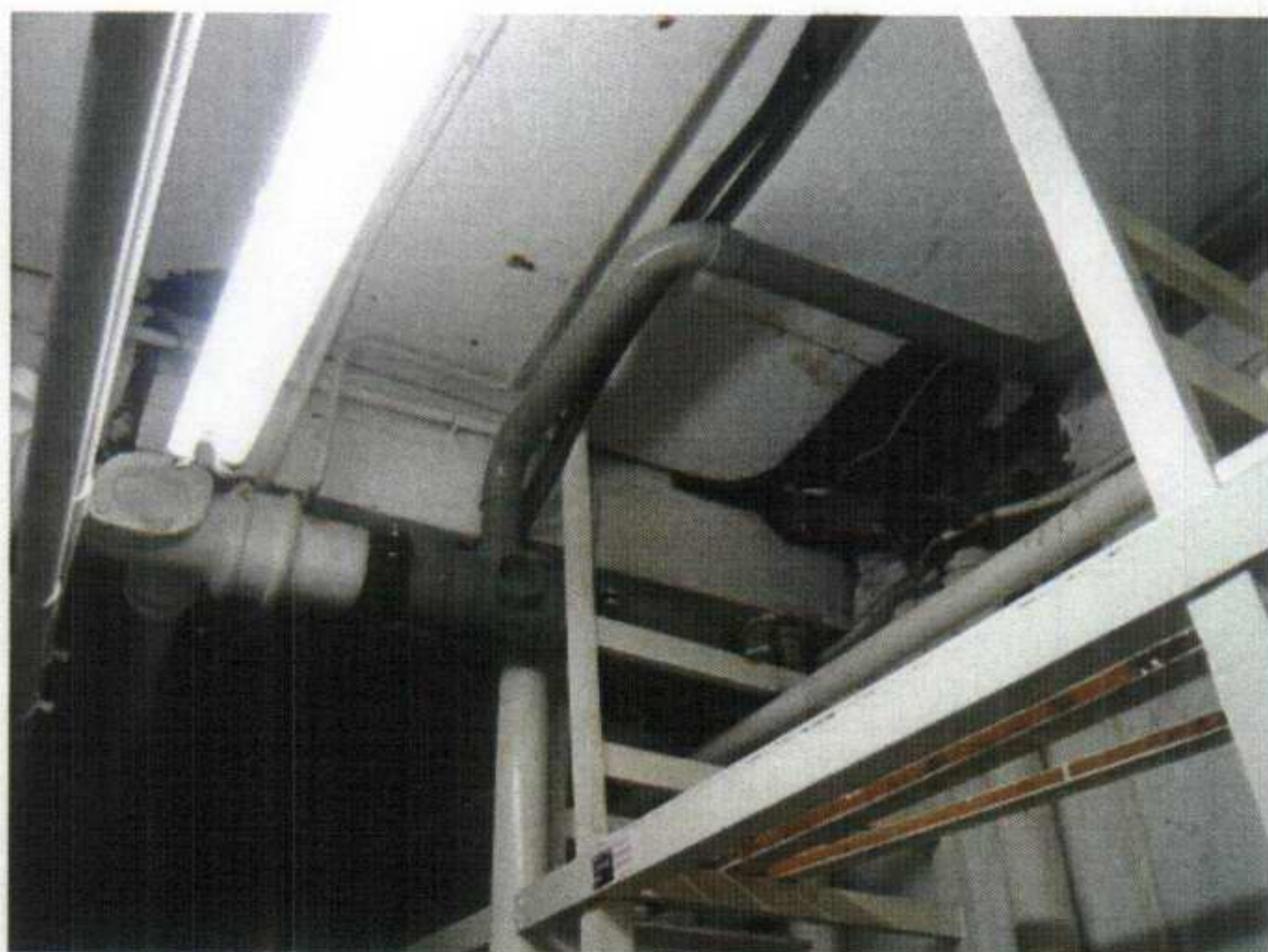
Figure 19 Room B22 Extensive ducts and pipes to be re-ordered and removed where possible.
