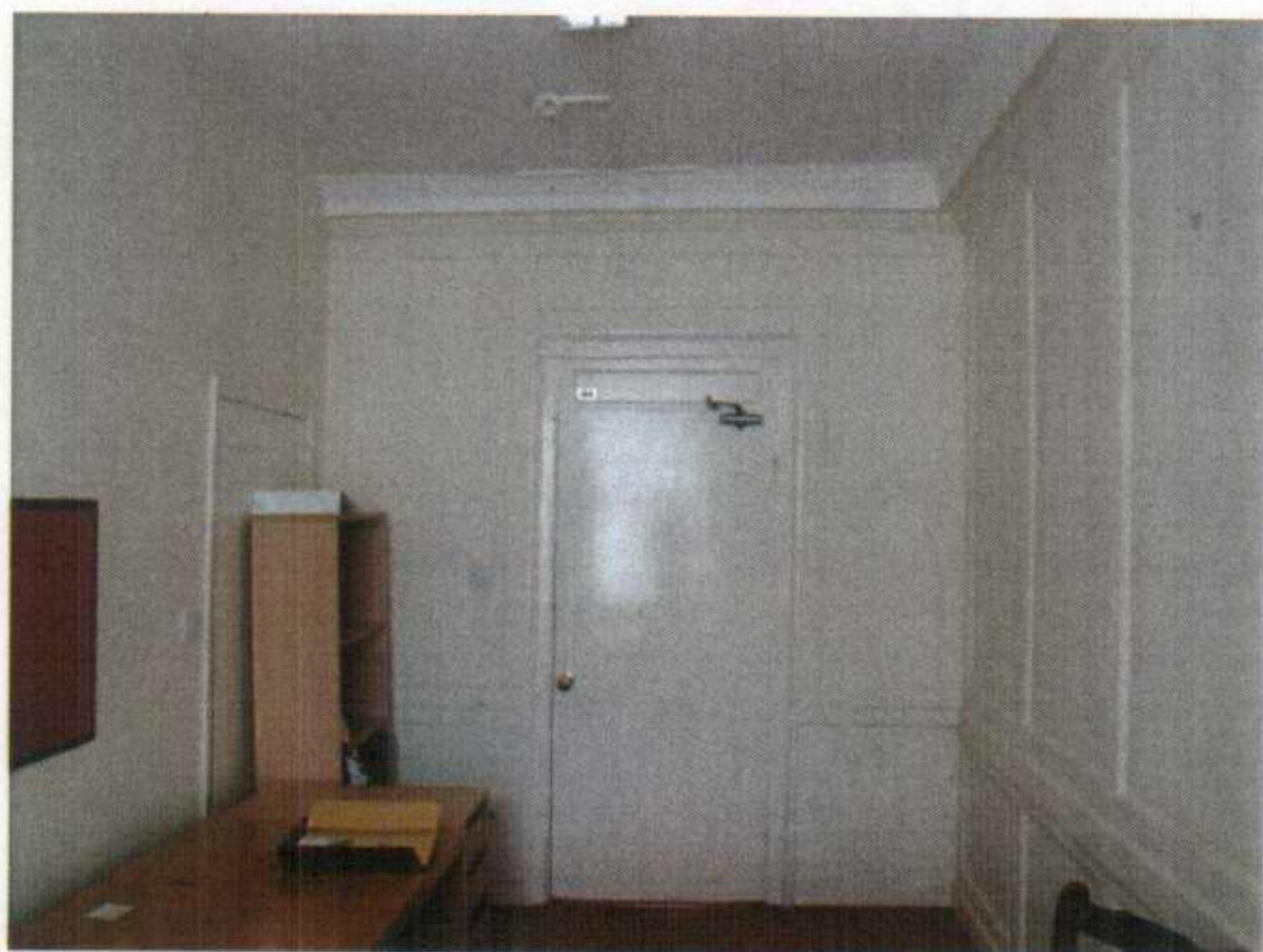
Figure 15 S12, part of existing modern partition to remain to form bathroom. No panels below dado on doorway wall and doorway altered. Modern panelling to wall on RHS of photo
