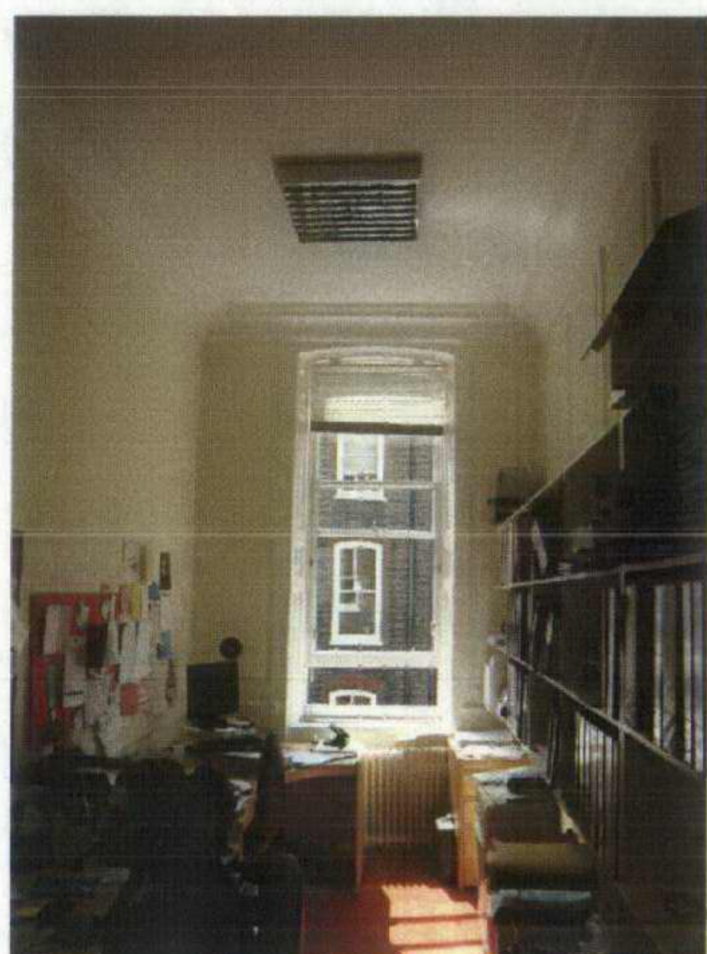
[no. 12] New partition to left of image - later cornice, not panelled
