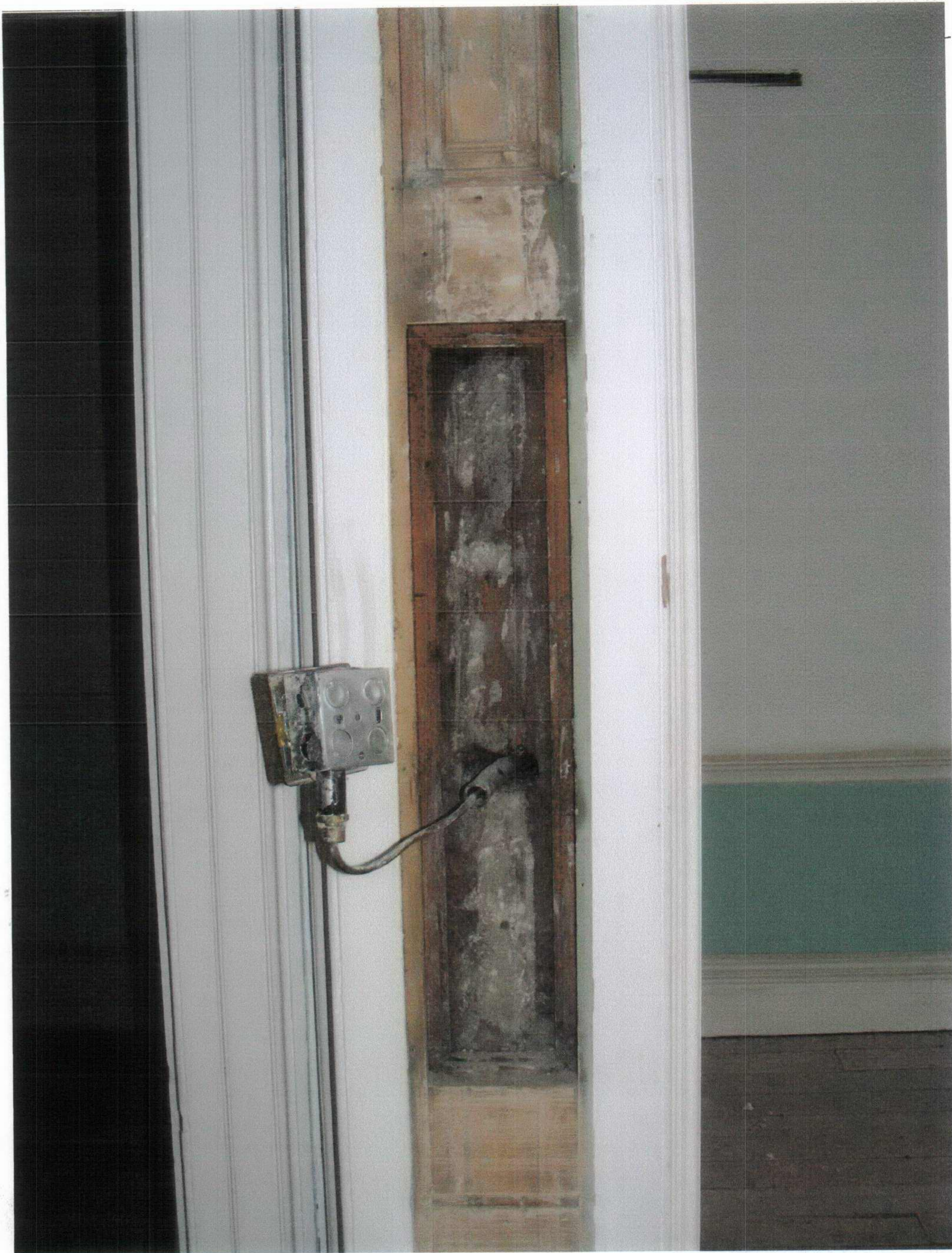
REPAIRS TO AREHWAY
