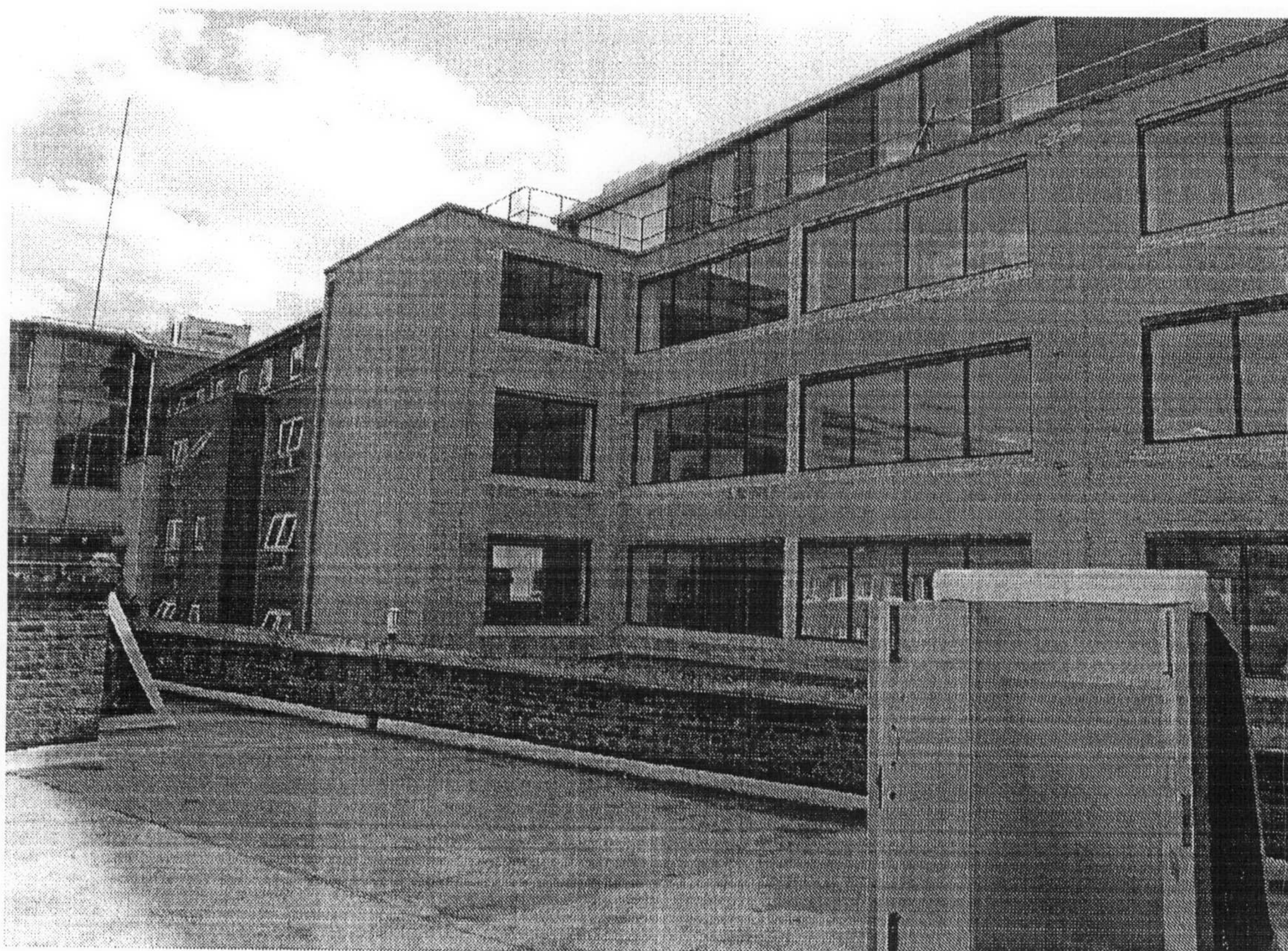
view of rear of 15-19 Kirkby Street from roof level
