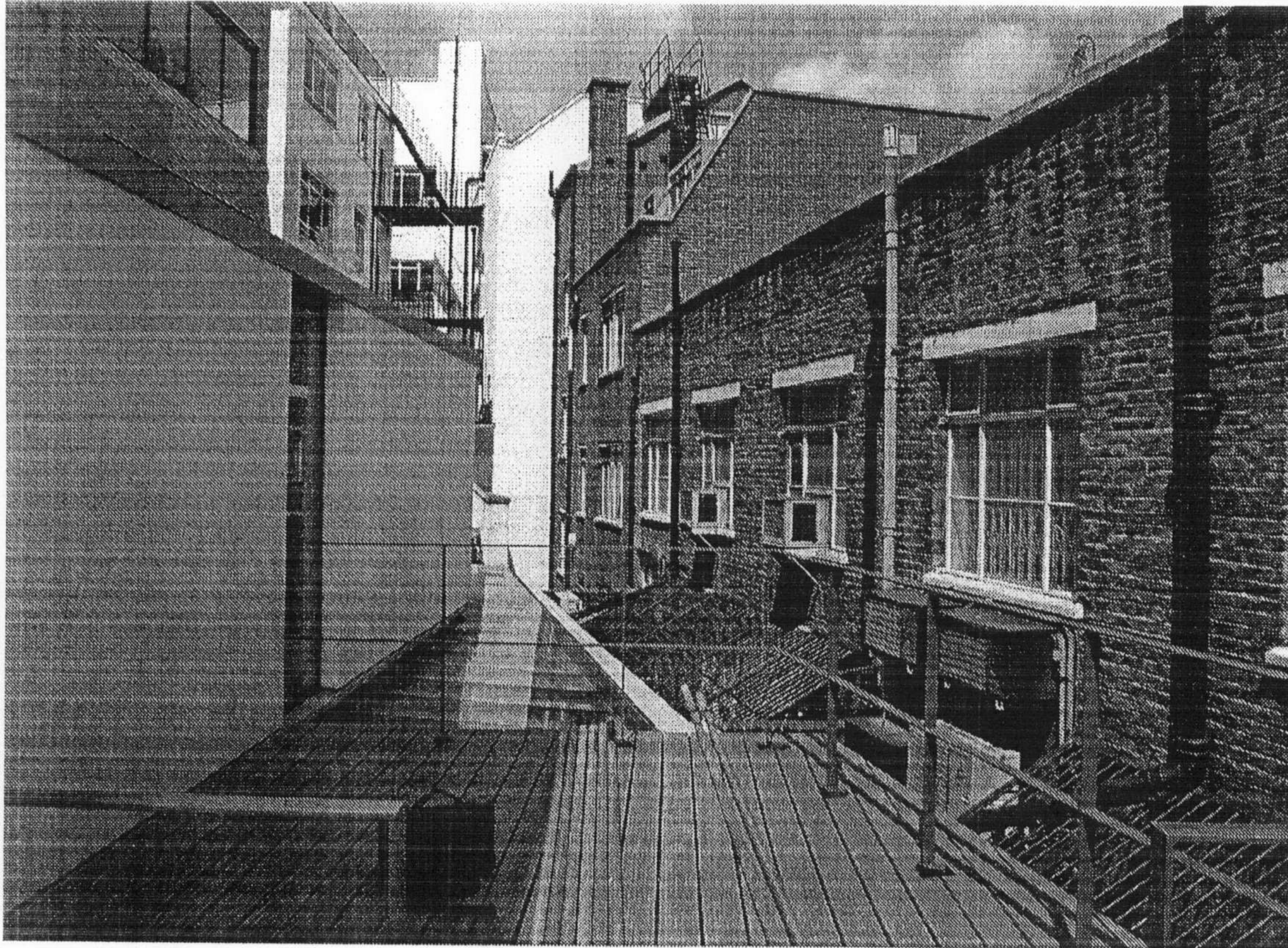
view of proximity of rear extension to Kirkby Street
