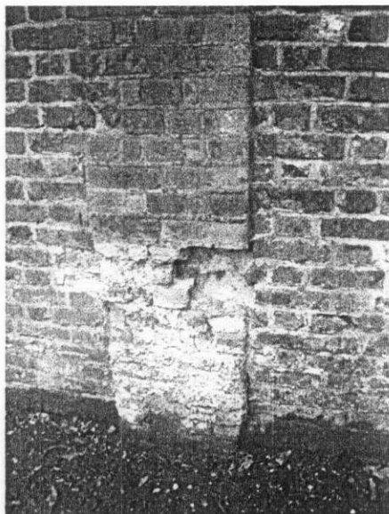
11. Repair existing pier, piece in missing brickwork and repoint.
