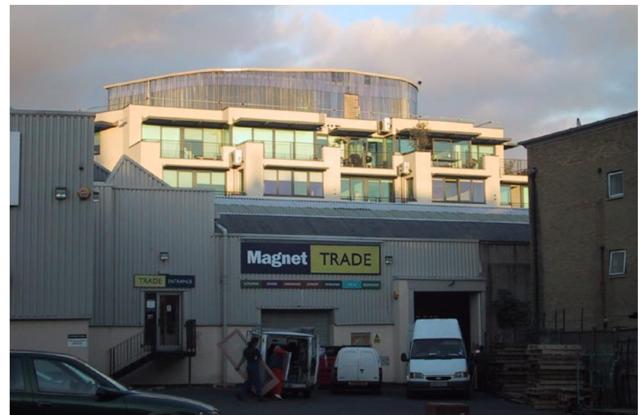
Fig. 2 View of 55 Holmes Road from Cathcart Street showing the existing plant room on the roof.
