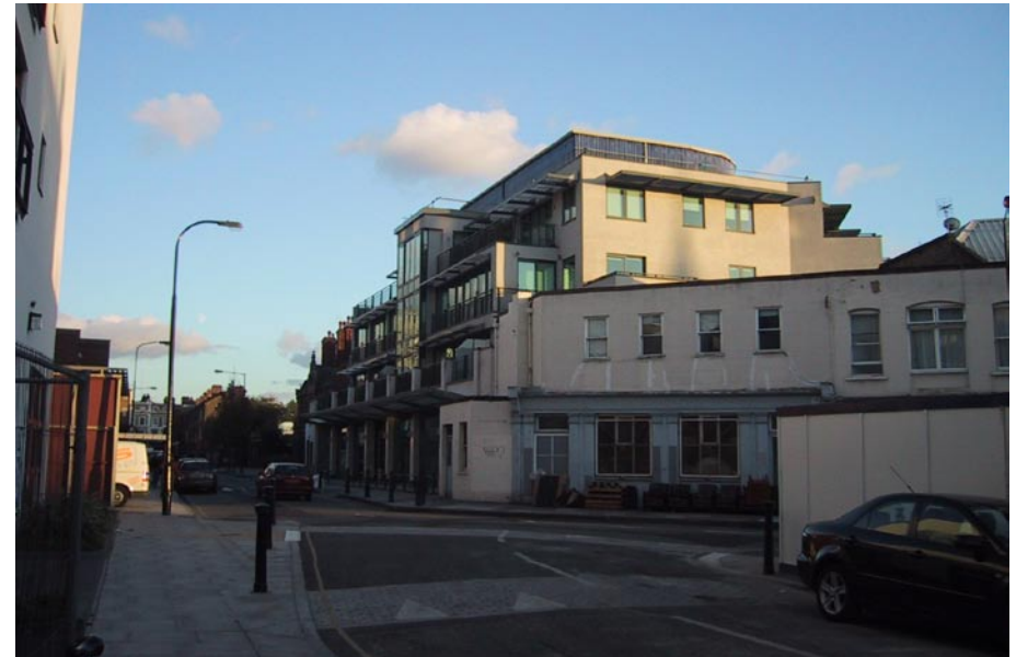
Fig. 1 View of 55 Holmes Road from Holmes Road showing the existing plant room on the roof.
