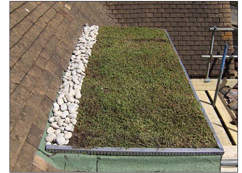
Sedum Roof – on un-accessed roof areas
