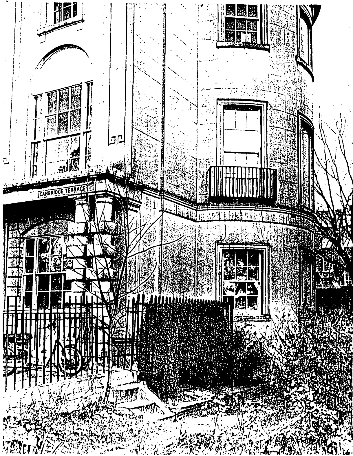
EXISTING APSE END TO NO. 1 CAMBRIDGE TERRACE.
