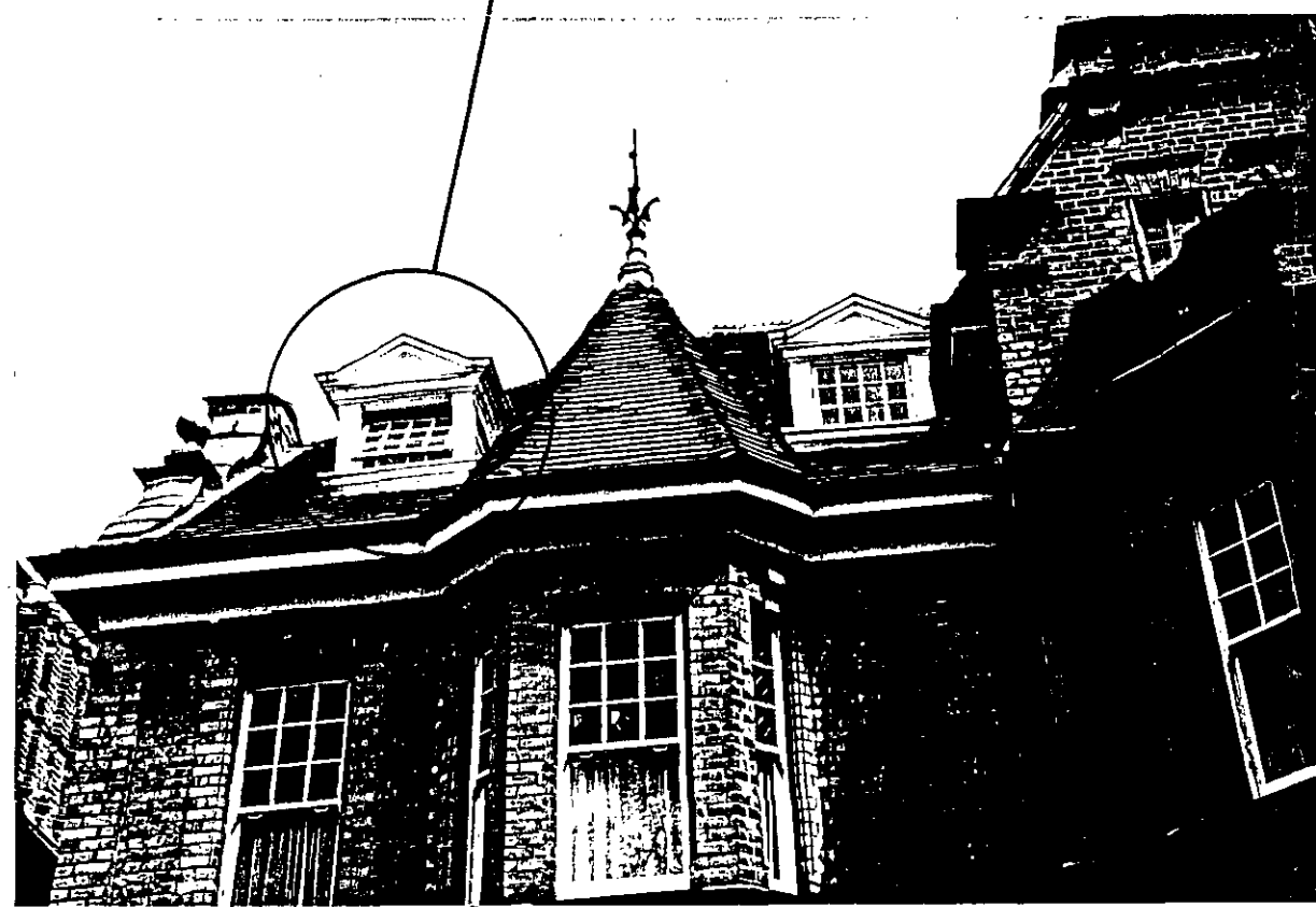
New dormer windows follow the model for the area.
