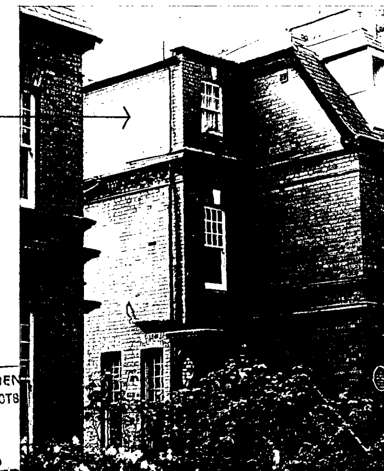
No 5 WELL RD.
