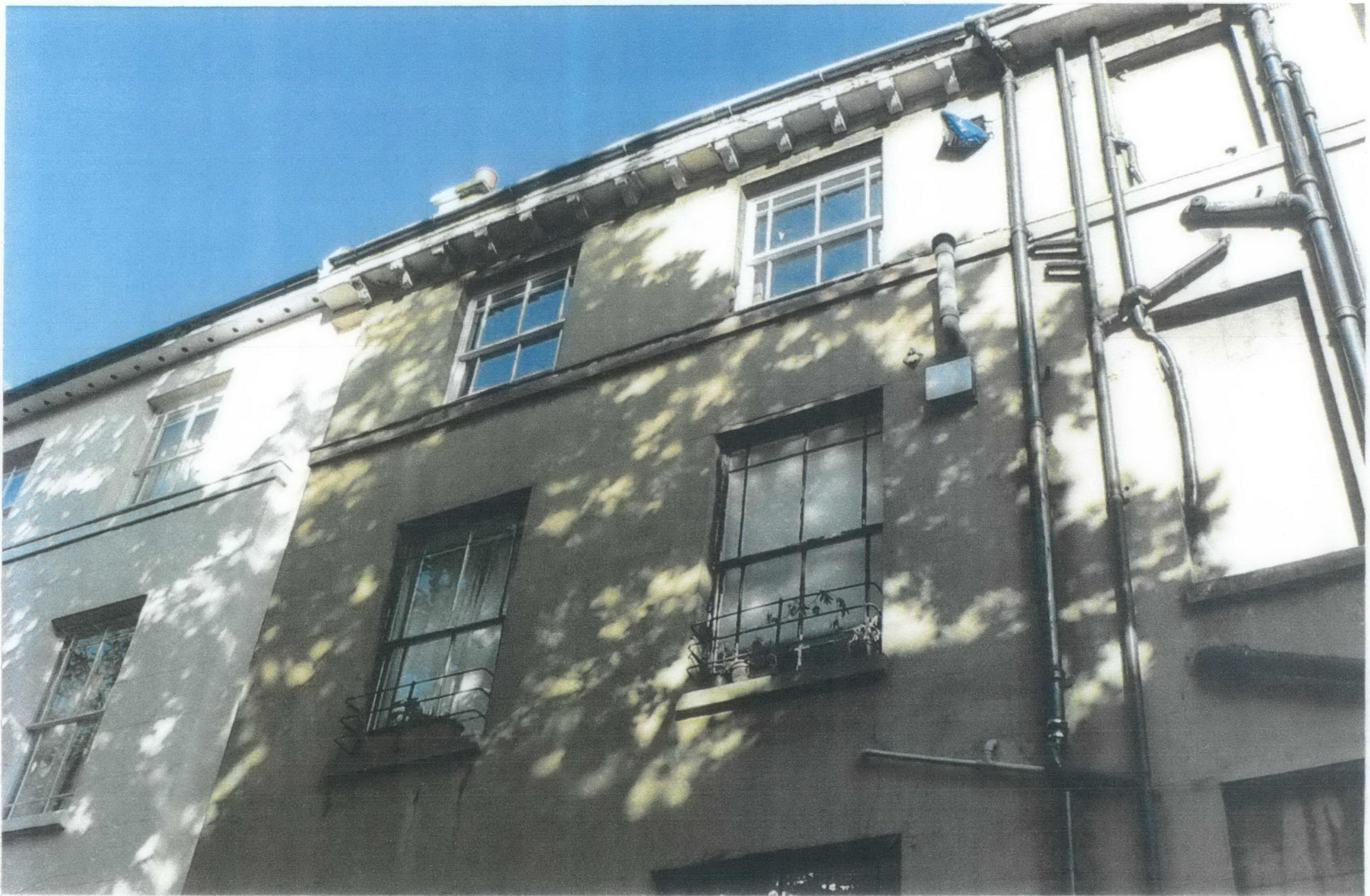
PROPOSED NEW WINDOWS, SECOND FLOOR, 17 REGENTS PARK ROAD, NW1 7TL REAR ELEVATION AS EXISTING
