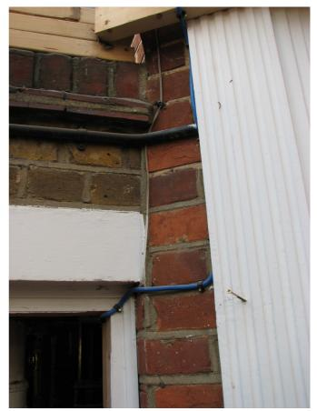
Existing ground f bor extension abutts the feature red bricks with a vertical joint. It is not bonded to the main house and hides the return brick.
