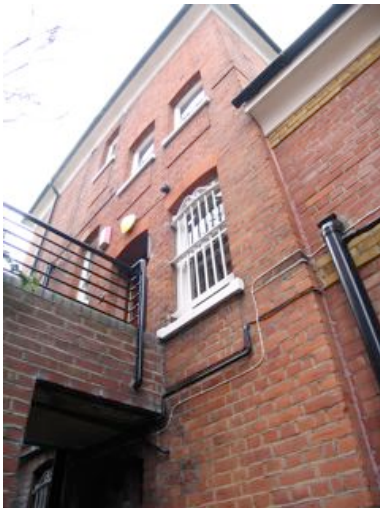
staircase and existing doorway to be returned to a timber sash window to match the window immediately to the right
