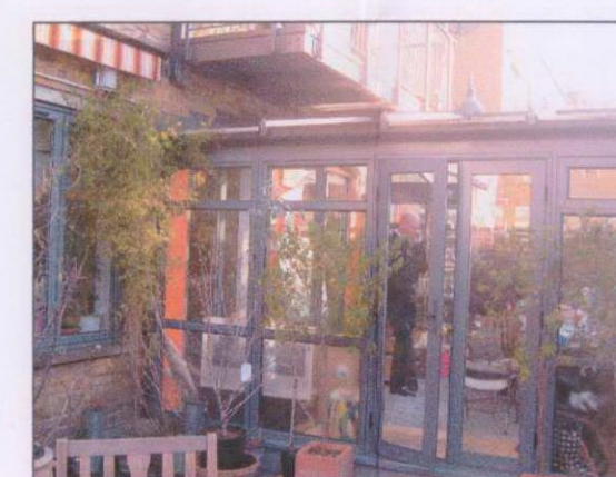
FIRST FLOOR REAR CONSERVATORY
