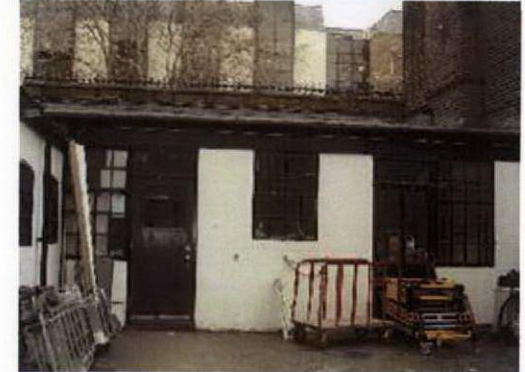
Existing workshop (to be demolished) looking North West
