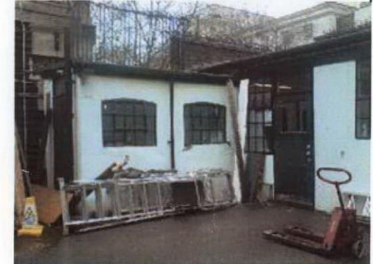
Existing workshop (to be demolished) looking West
