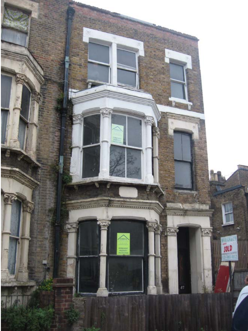
IMAGE 1 - SHOWING EXTERIOR ELEVATION OF EXISTING BAY WINDOWS
