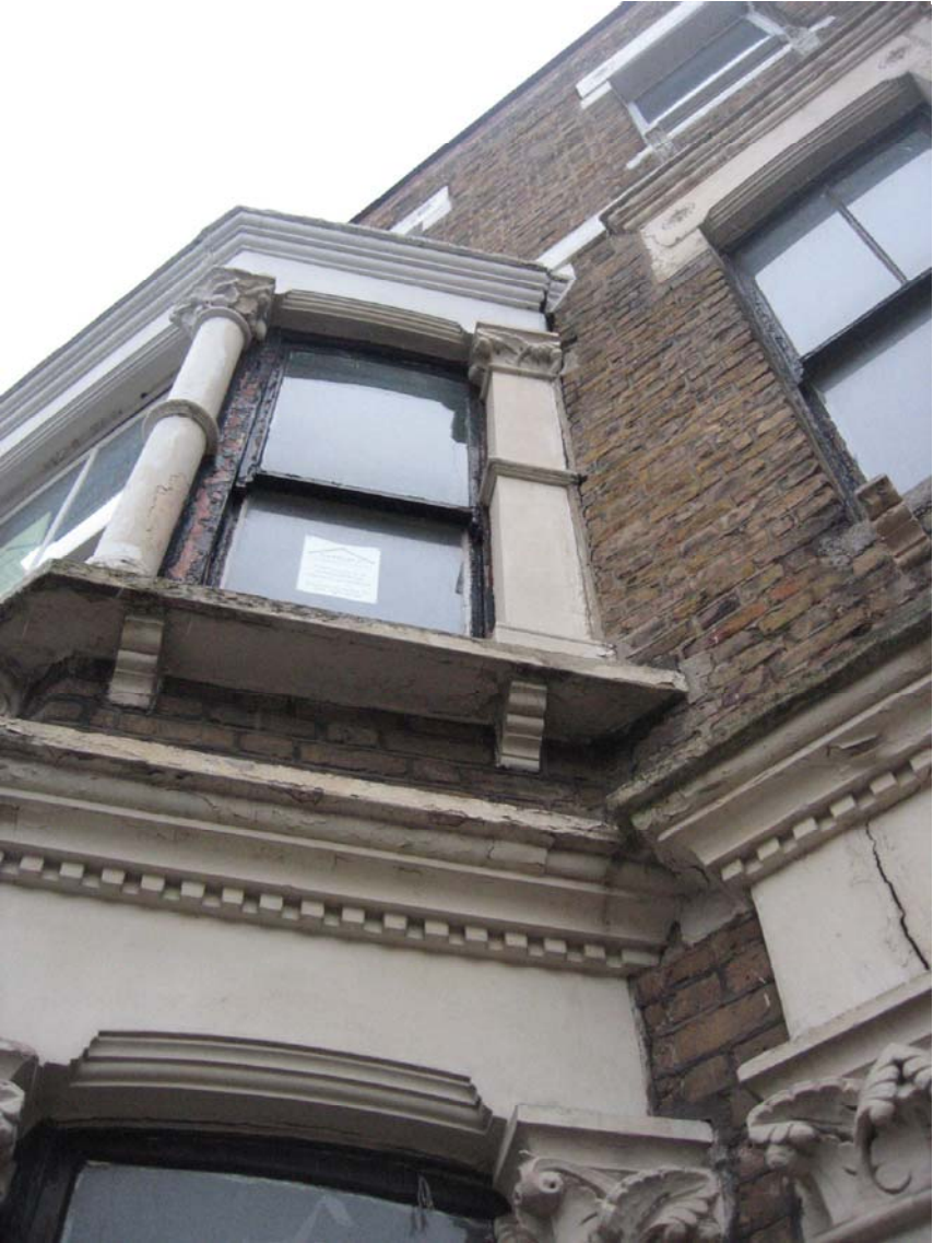
IMAGE 3 - SHOWING EXTERIOR ELEVATION OF EXISTING BAY WINDOWS
