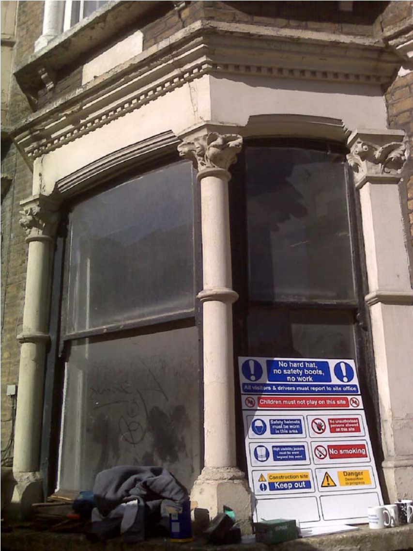
IMAGE 2 - SHOWING EXTERIOR ELEVATION OF EXISTING BAY WINDOWS
