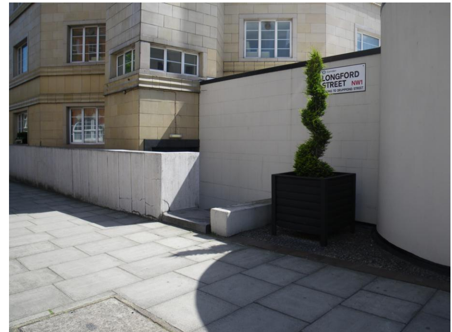
Figure 5.9: Photo of Hotel Fire Escape (docking areas to be at either side of this access)
