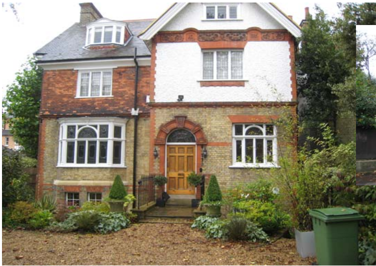
Front Facade - Keats Grove
