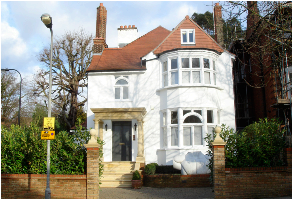
No. 1 Hollycroft Avenue Front View
