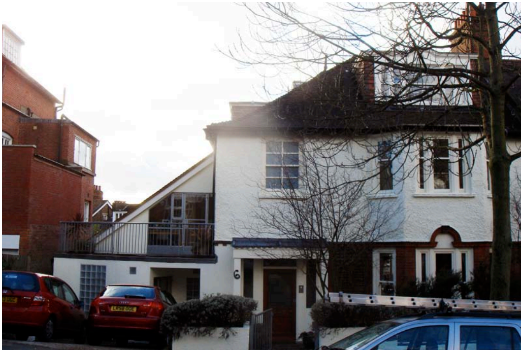
No. 6 Hollycroft Avenue Front View
