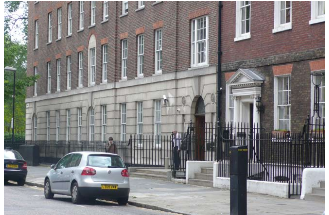
Photo 2 - View of John Street Ground Floor Elevation
