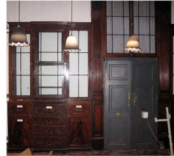
Wall cabinets (A & B) with safe in chimney breast and glazed cabinet above
