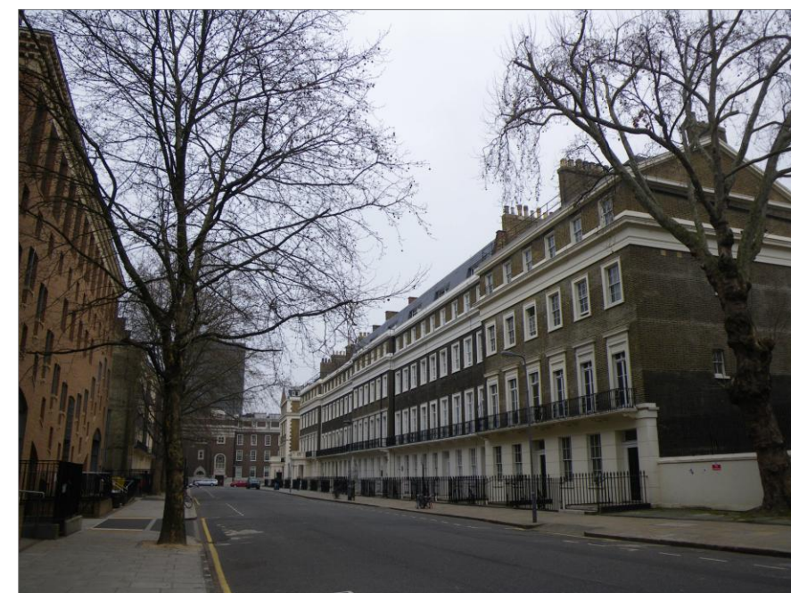
Figure 5.9: View of no's 1-12 Taviton Street, viewed from the site, looking north along Taviton Street
