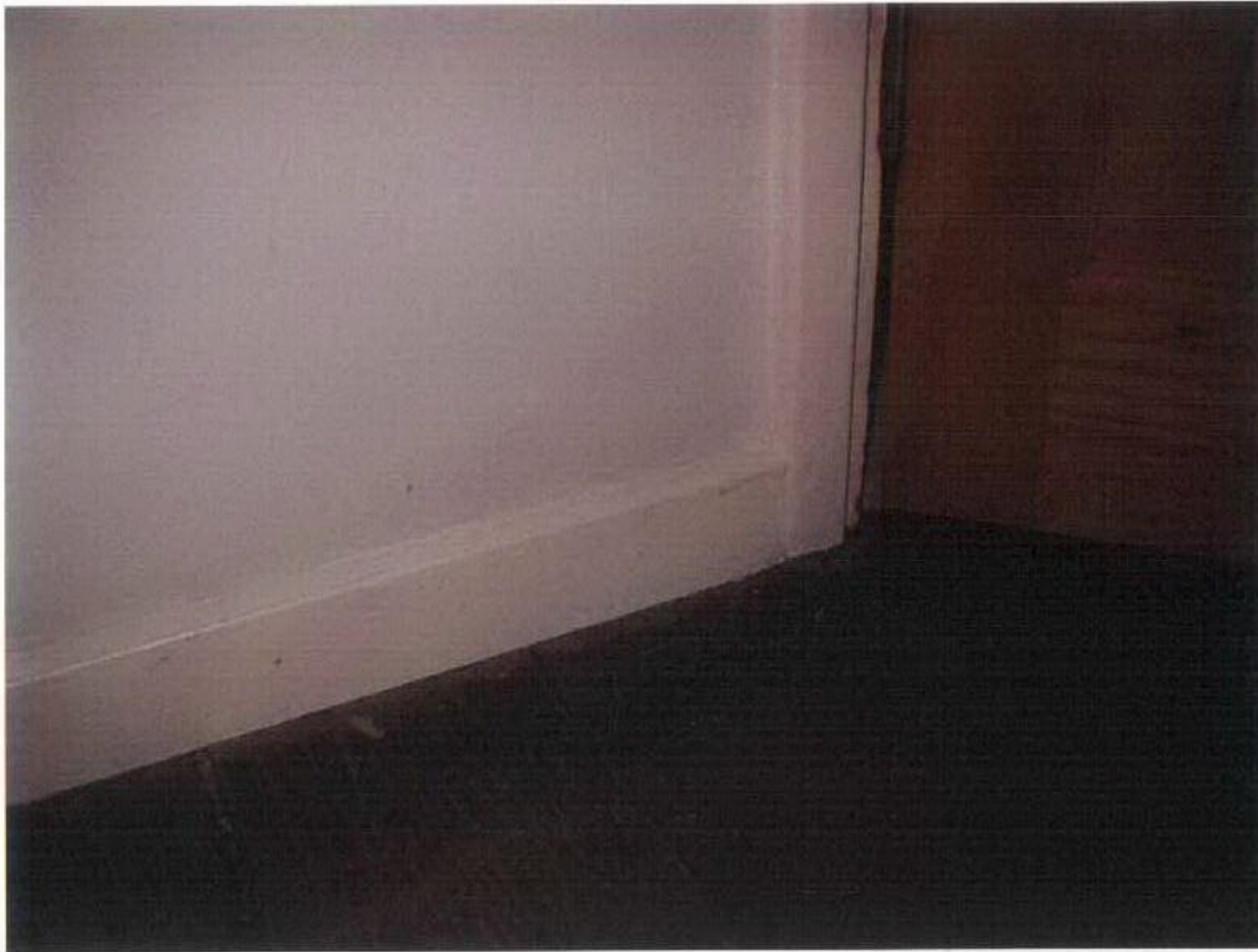
Photograph No. 17 – Skirting board to north wall Bedroom - 29 Buckridge Building
