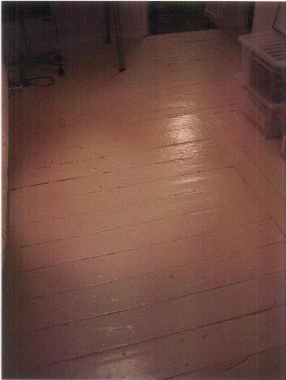
Photograph No. 7 29 Buckridge Building
