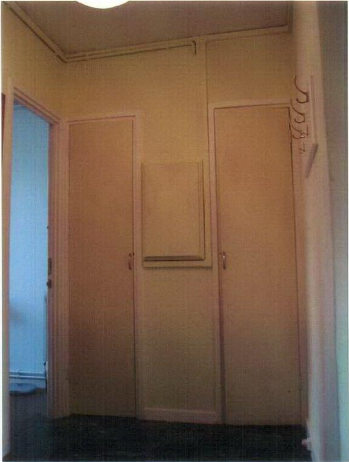
Photograph No. 5 29 Buckridge Building
