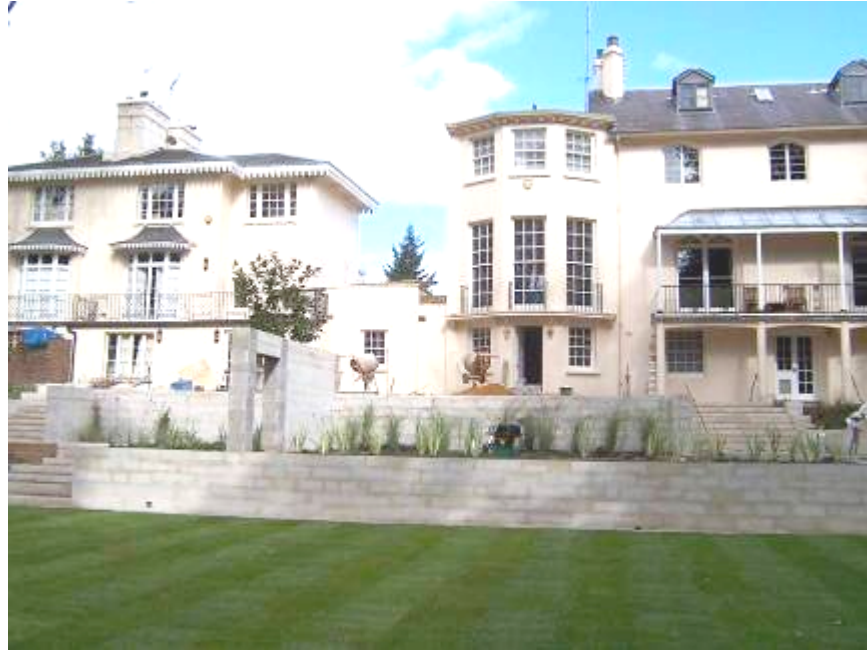
PHOTOGRAPH 3: GENERAL VIEW OF TERRACES UNDER CONSTRUCTION
