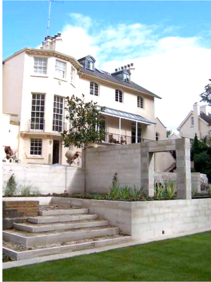
PHOTOGRAPH 1: WALL UNDER CONSTRUCTION
