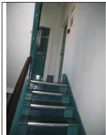
Fig. 2.51.1– View of Wall 1/2
