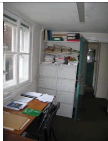
Fig. 3.2.3 – View of Wall 2/3
