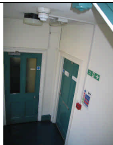
Fig. 2.51.2 – View of Wall 2/3
