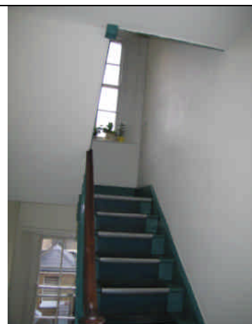
Fig. 2.52.3 – View of Wall 3/4
