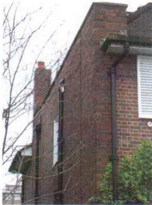
Existing quoin and parapet detail
