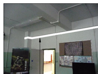
U HIGH LEVEL TRUNKING UNDER BEAM
