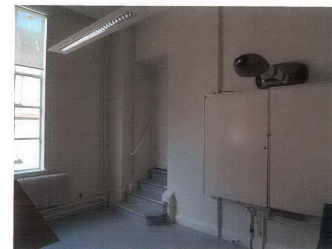
View from Classroom (Room 23A)
