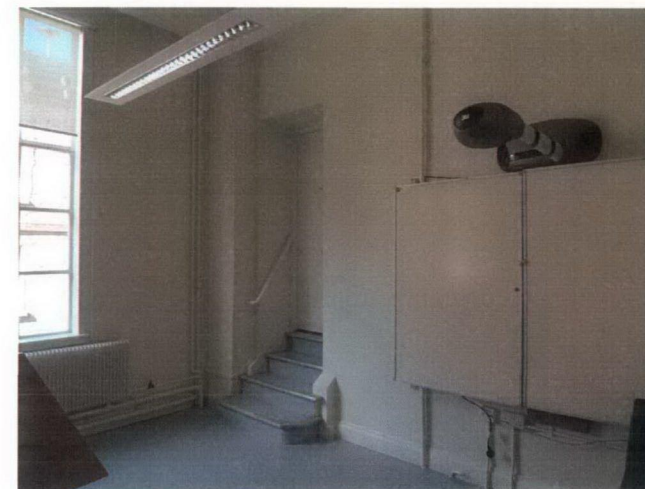
View from Classroom (Room 23A)
