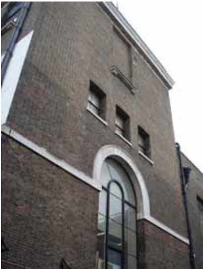
Fig.2 – The North Wing West Elevation - the end of the Arched Room
