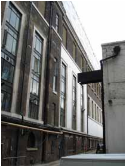
Fig.1 – The North Wing North Elevation
