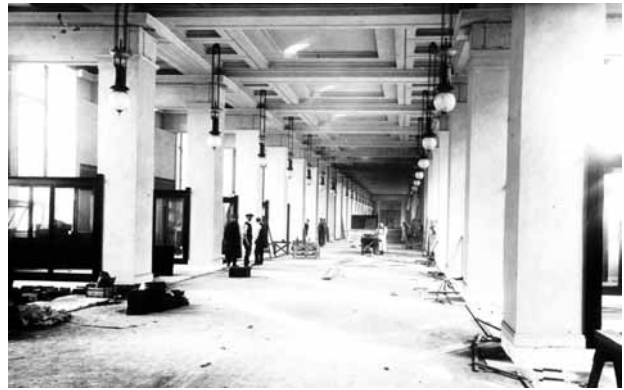
Fig.22 – The Hotung Gallery shortly before its completion showing the pendant electric lights
