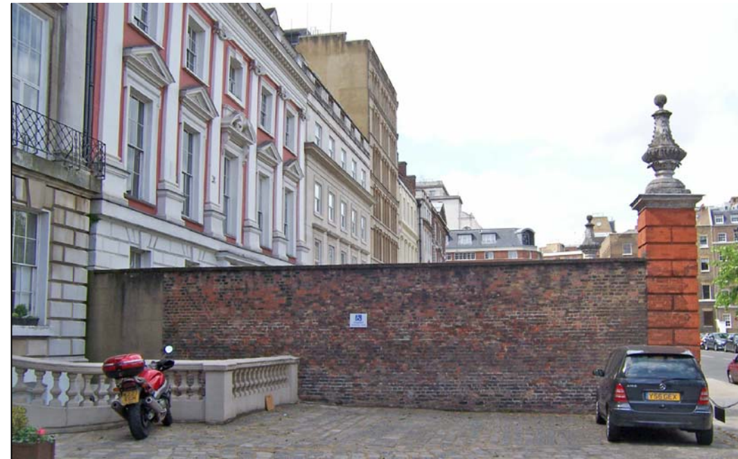
Photograph of the South Wall, Looking North, as Existing
