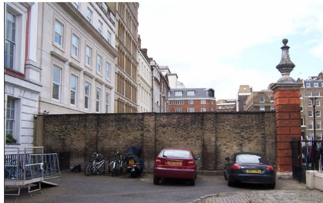
Photograph of the North Wall, Looking North, as Existing
