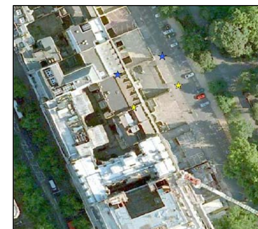
Aerial views of the site. South wall marked with yellow stars, north wall marked with blue stars.
