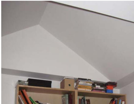
SECOND FLOOR BEDROOM: raised ceiling level into roof void
