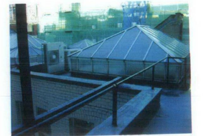
Existing skylight destined for removal
