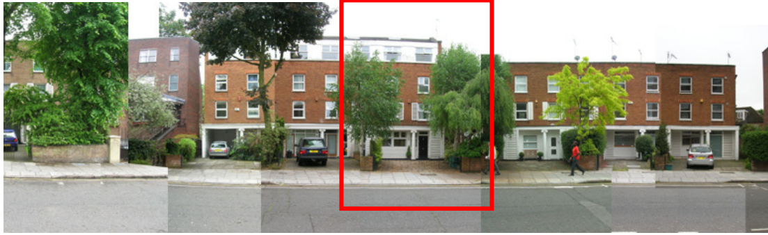
Front elevation and adjacent properties (Image 3.1)
