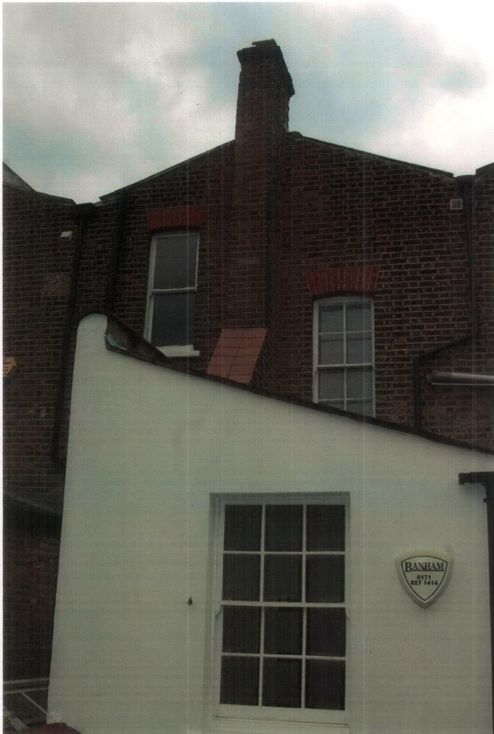
Existing shallow pitched roof to be replaced by flat terrace
